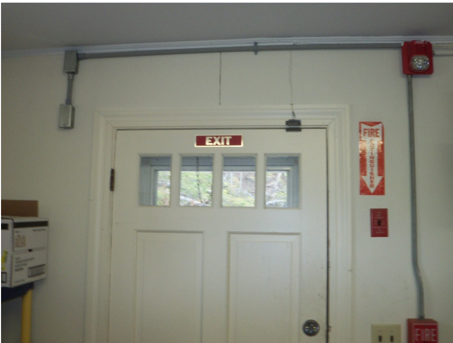
Photo CC-6: Kitchen Egress Lighting and Fire Alarm example
