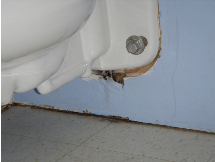
Photo GSC21: Water damaged gypsum board at Toilet
