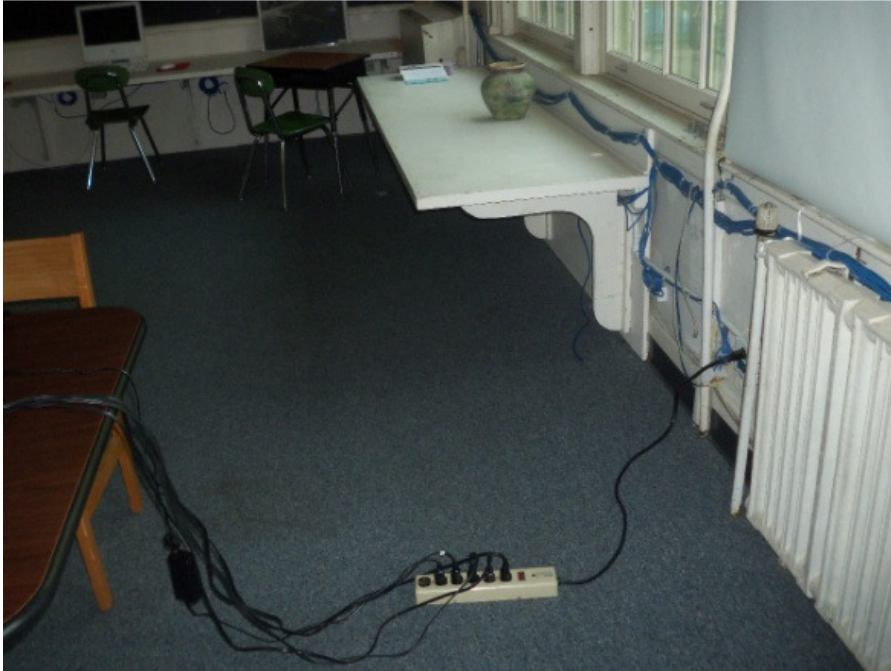
Photo PS-5: Exposed wiring and inadequate convenient general purpose outlets
