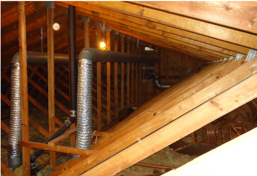
Photo CC5J: Exhaust systems serving the locker room.
