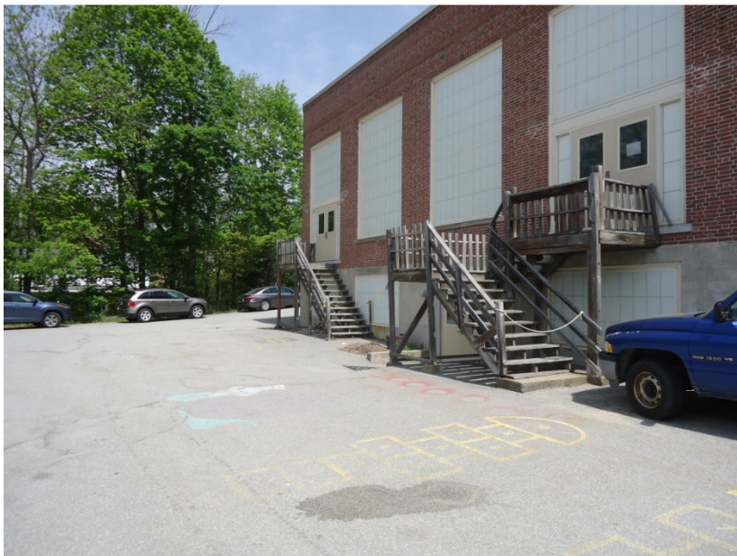
Photo PS3C: Exterior egress stairs at the rear of the building and serving the gymnasium are not code compliant.
