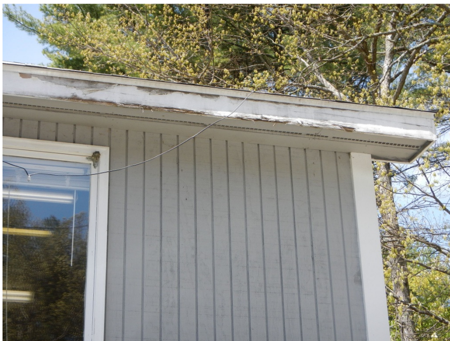
Photo GSC32: Deteriorated wood fascia trim Loose snow melt wiring
