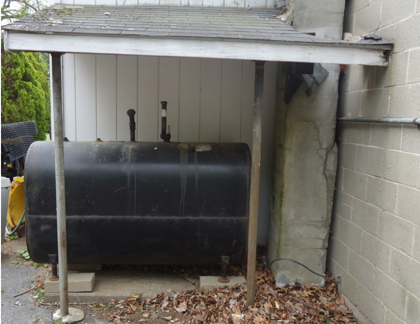
Photo CC5I: Existing Fuel/Oil Storage Tank with Supply Line. Also note the condition of the chimney directly adjacent.
