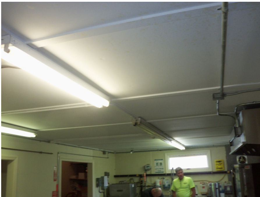
Photo CC-4: Exposed lamps
