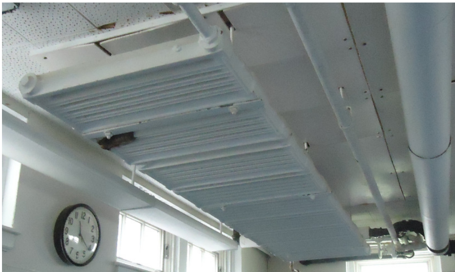
Photo PS4B: Existing Radiator Which Has Been Repaired.
