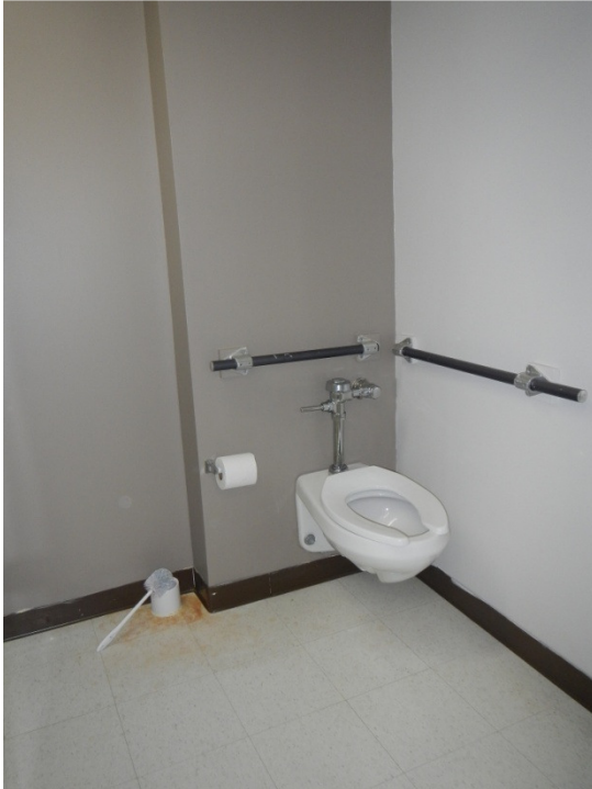
Photo GSC19: Non-Compliant Handicap Accessible Toilet
