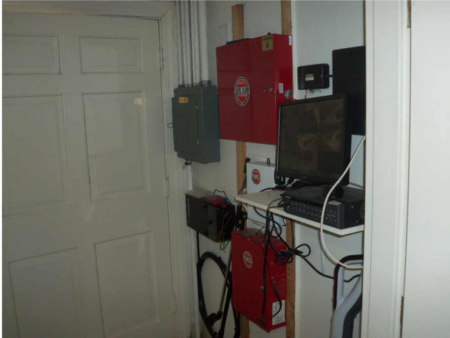
Photo CC-3: Improper placement of electrical equipment
