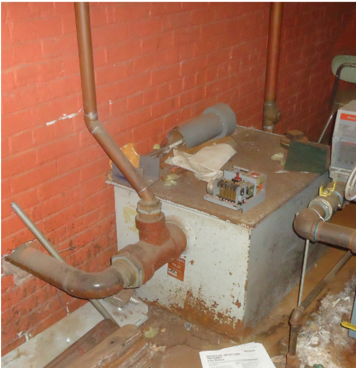
Photo PS3C: Existing Grease trap located in boiler room adjacent to kitchen.
