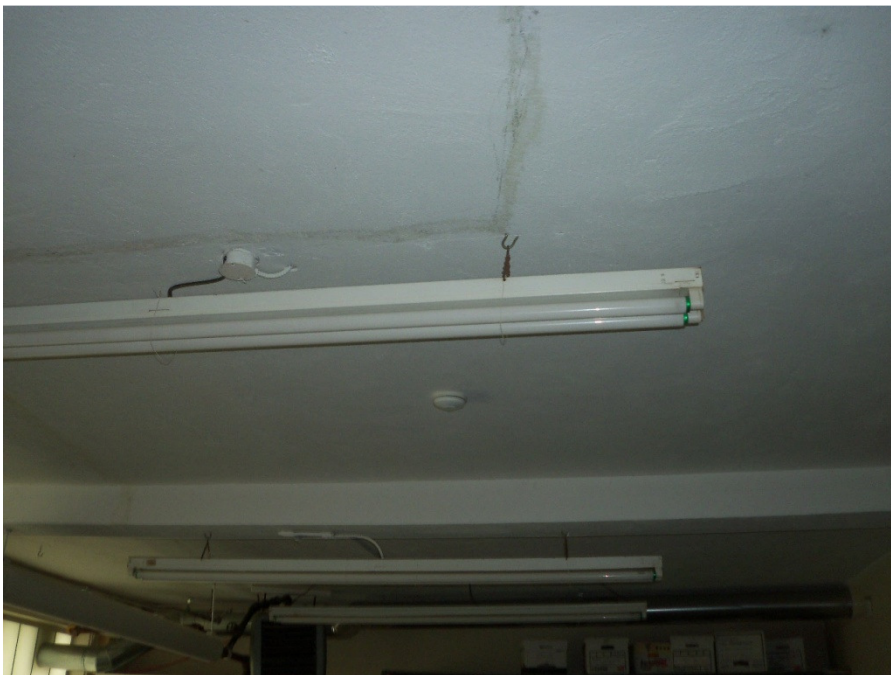
Photo PS-2: Exposed lamp fixture
