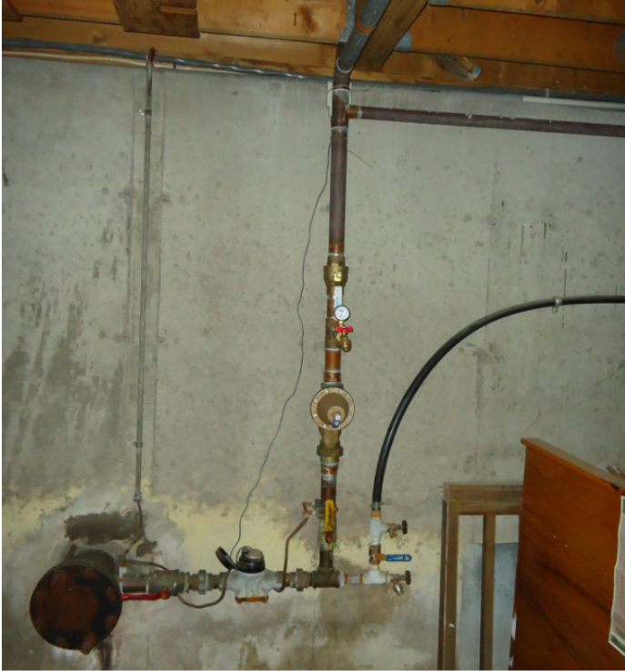
Photo CC3A: Existing water service to the building
