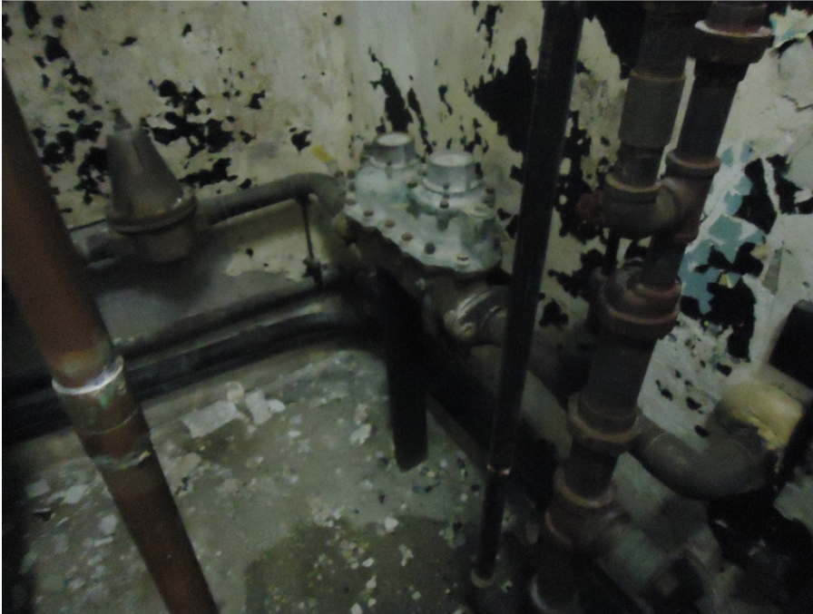
Photo PS3A: Incoming 2" Water Service with pressure reducing valve and backflow prevention.
