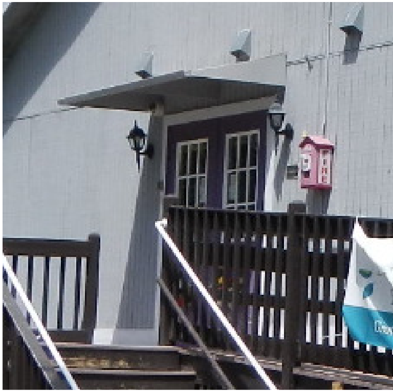
Photo GSC6D: Restroom Exhaust Terminating Over Entry of Building
