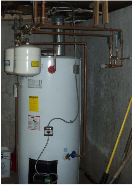
Photo CC3C: Existing domestic water system showing water heater, expansion tanks and temperature mixing devices.
