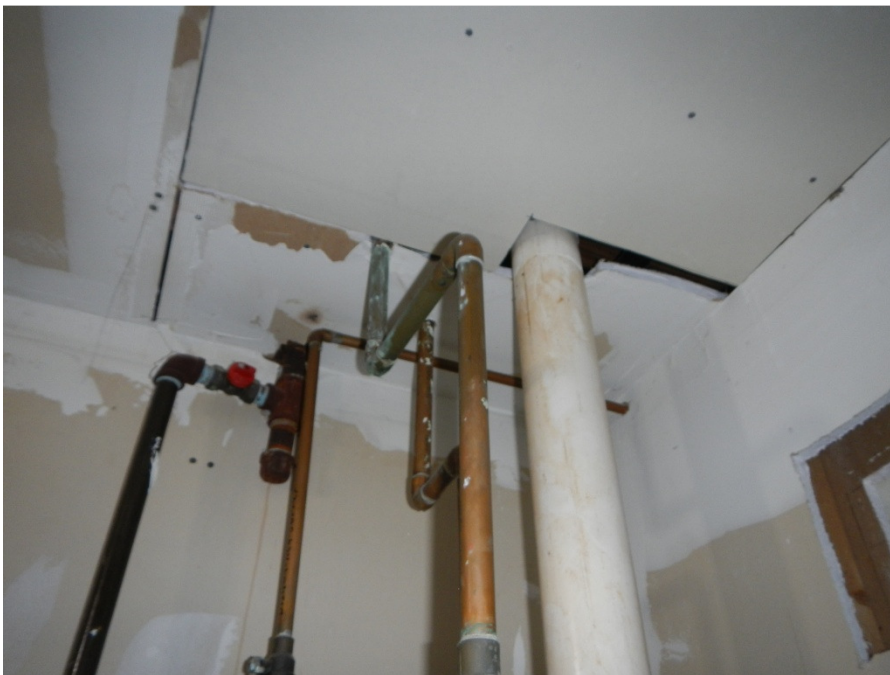
Photo GSC30: Unprotected openings in fire-rated ceiling construction
