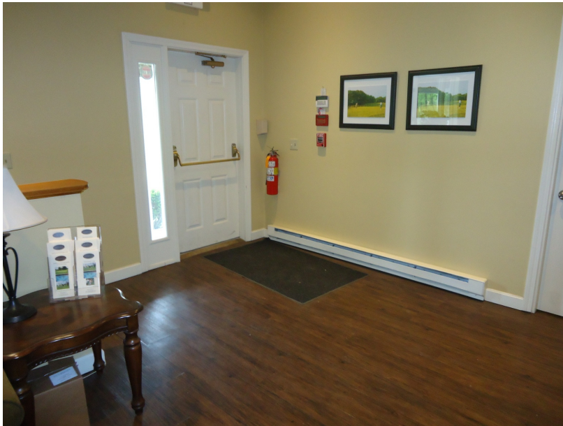
Photo CC6A: Main entrance to facility lacks an entry vestibule, resulting in energy loss during heating/cooling cycles.
