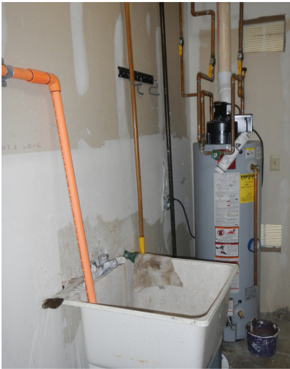
Photo GSC3B: Existing Domestic Water Heater. Note High and Low Openings into Adjacent Space for Combustion Air.
