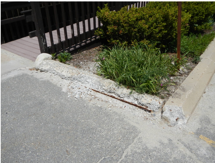
Photo GSC12: Deteriorated concrete curb near Main Entrance.
