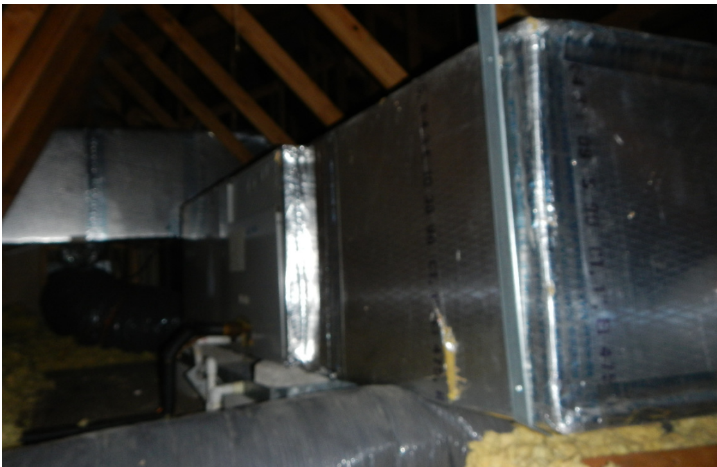
Photo GSC6C(2): Split system air handling unit located in the Attic.
