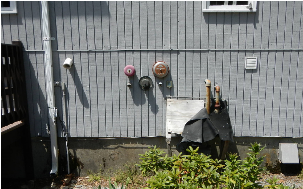
Photo GSC5A(2): Existing Gas Meter Enclosure. Picture also shows Fire Department Connection, Alarm, Domestic Water Heater Vent, Dryer Vent and through wall intake louver.
