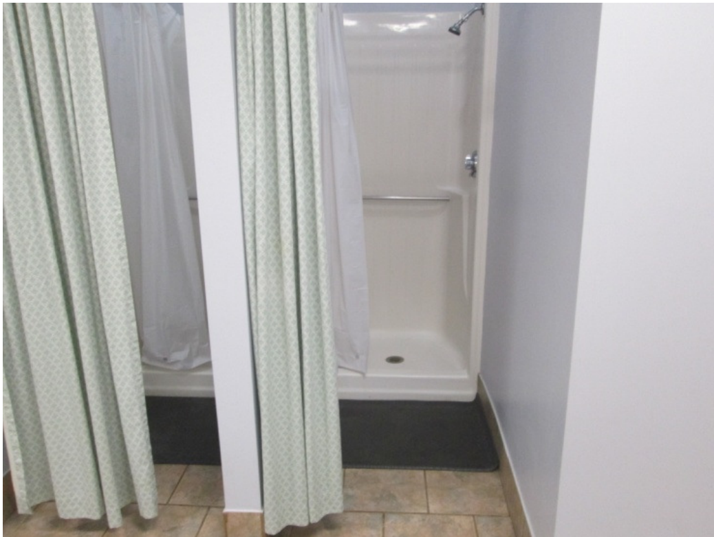
PhotoCC4D: Locker rooms lack numerous accessible features including accessible shower stalls and entrances.
