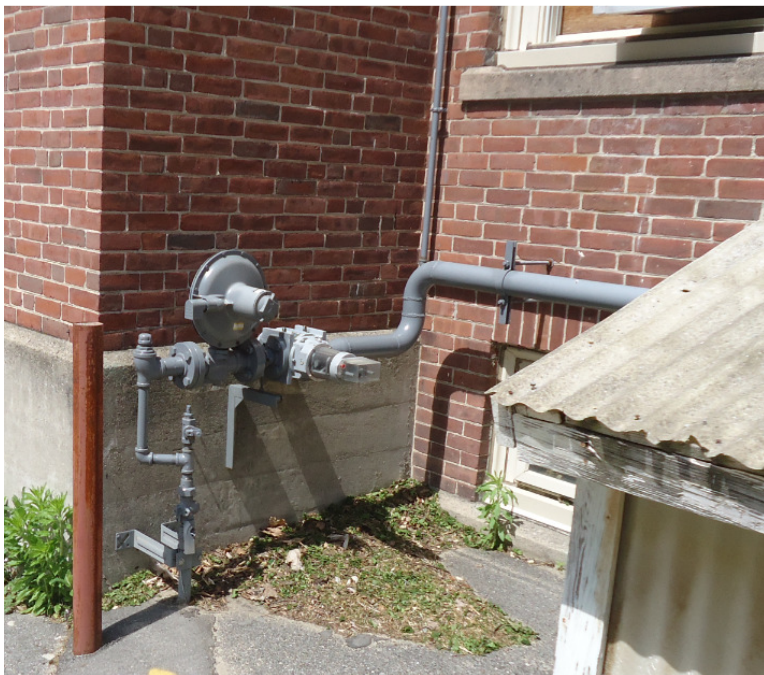
Photo PS3G: Existing Gas Service to the Building.
