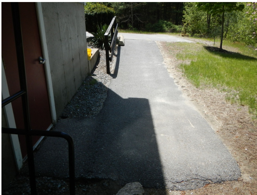
Photo GSC10: Non-Compliant accessible ramp to Lower Level
