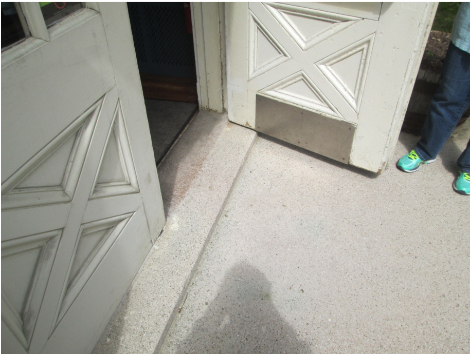
Photo PS4C: Designated accessible entrance door is heavy, lacks power assist, contains non-compliant threshold.
