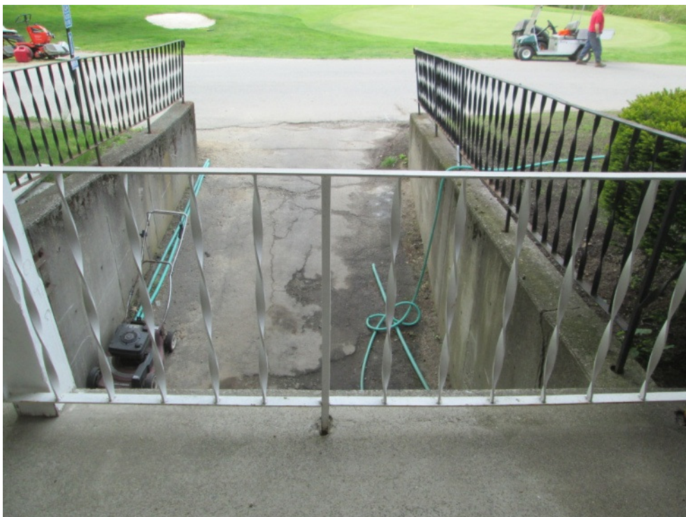
Photo CC3B: Fall hazards. Horizontal guard railing less than 42 inches in height. Spacing of vertical members exceeds 4 inches and allows passage of small child through railing.
