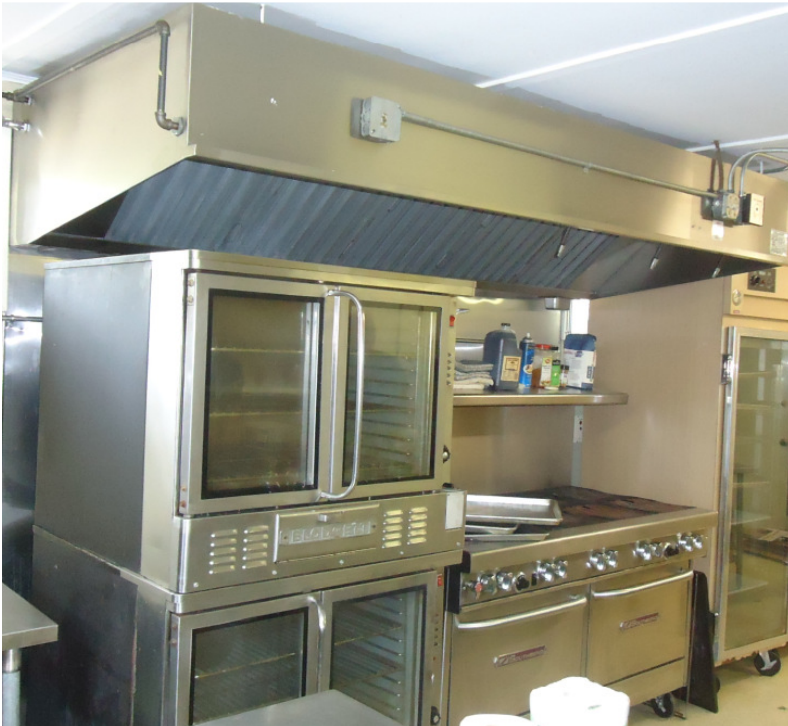
Photo CC5F: Type 1 grease exhaust system with fire suppression.
