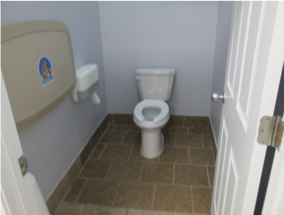
Photo CC4D: Toilet compartment lacks accessible grab bars and turning radius. Doors contain inaccessible knob hardware and lack lever handles.
