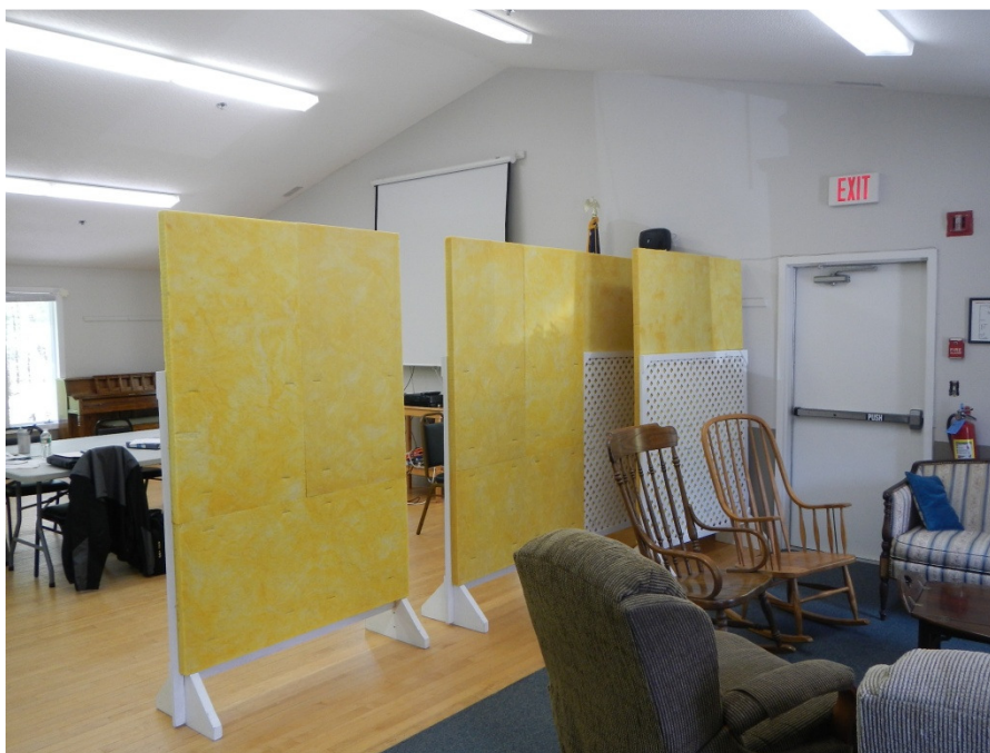
Photo GSC18: Temporary / Portable acoustical partitions in Meeting Hall
