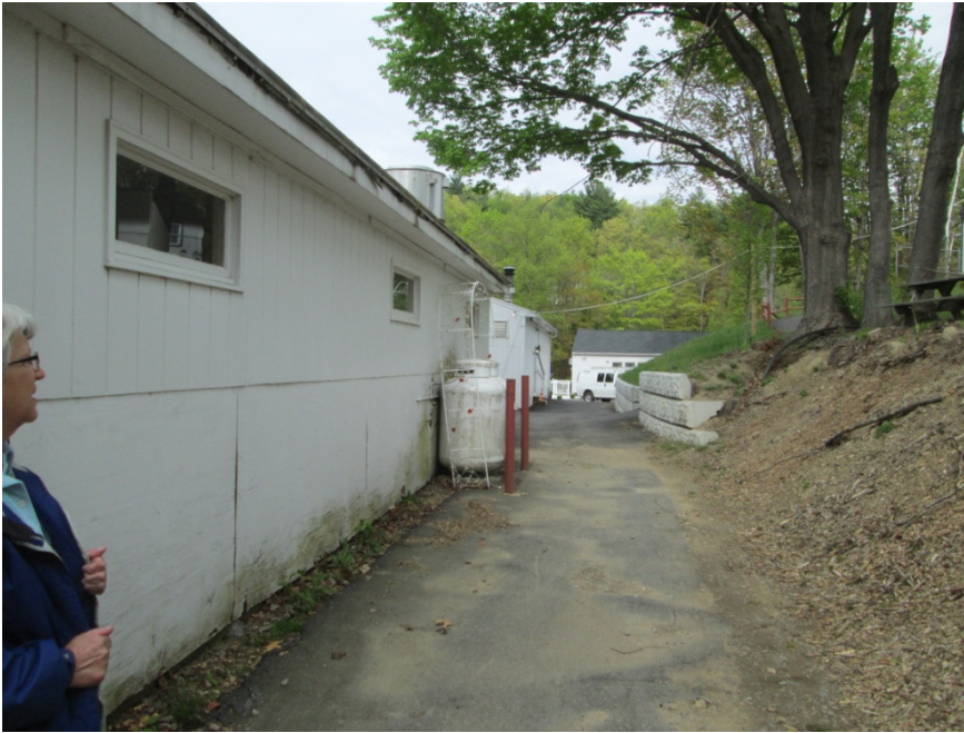
Photo CC7D: Deteriorated wooden siding at rear elevation. Hillside at rear limits expansion possibilities.
