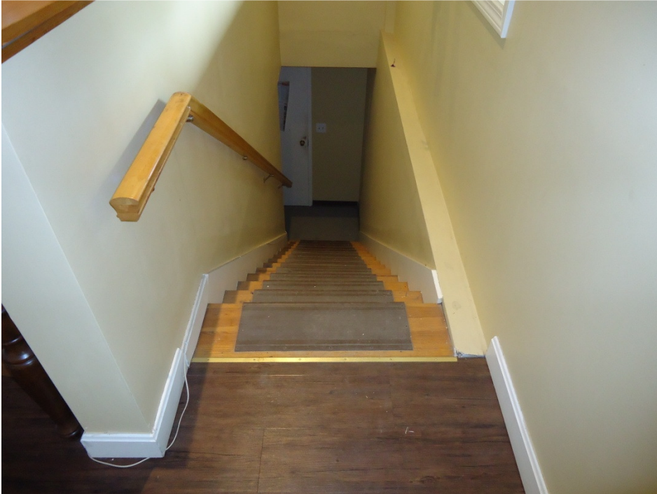
Photo CC10F: Existing stair to basement is 36 inches wide.
