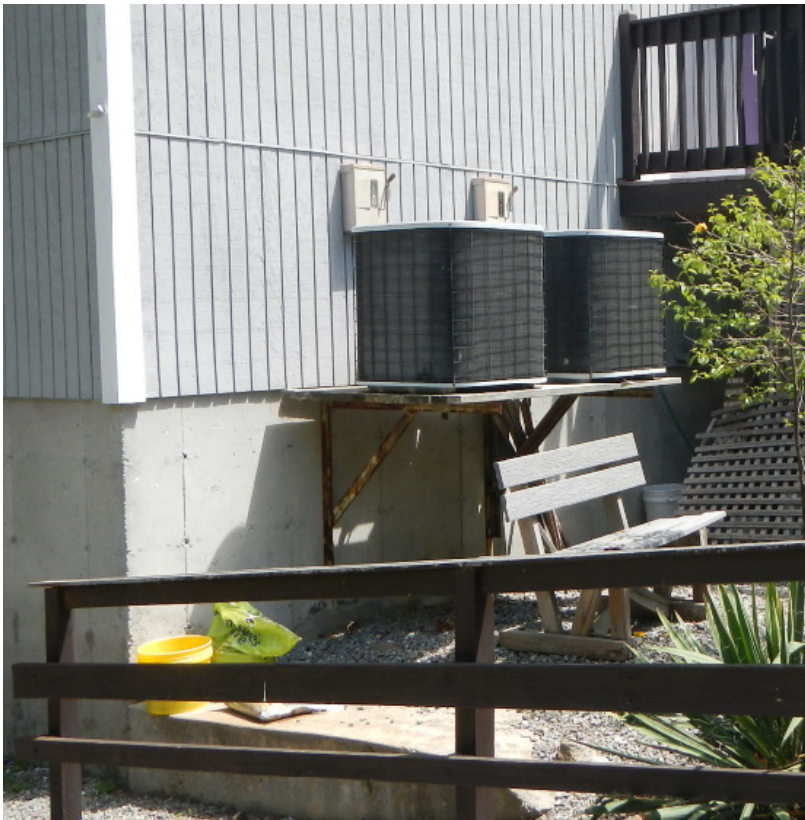
Photo GSC6C(1): Condensing Units located on Platform.
