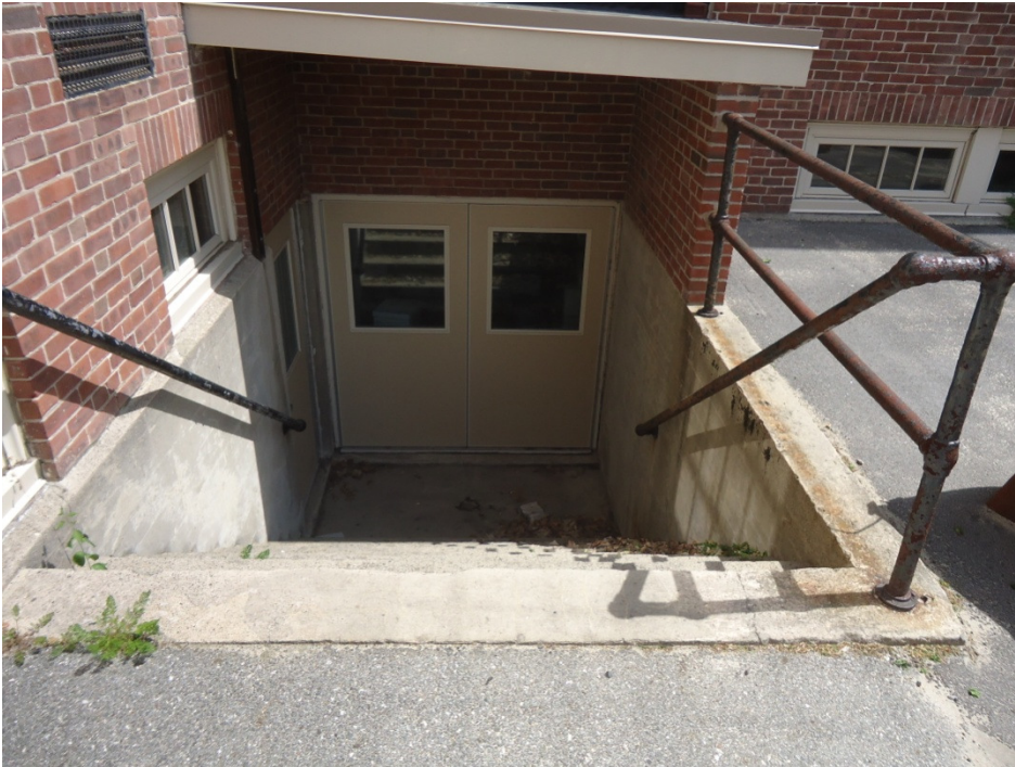
Photo PS3E: Non-compliant guard rails and handrails at stair.
