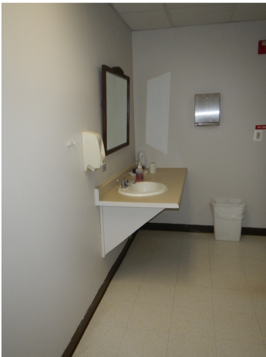
Photo GSC20: Non-Compliant Handicap Accessible Lavatory and Mirror
