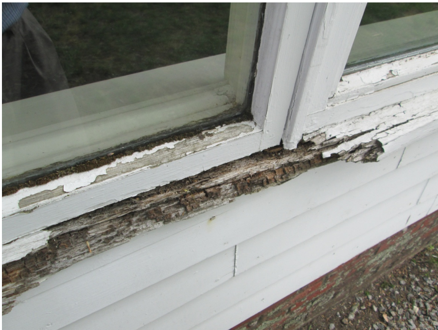
Photo CC7B: Deteriorated wooden window, sill and associated trim.
