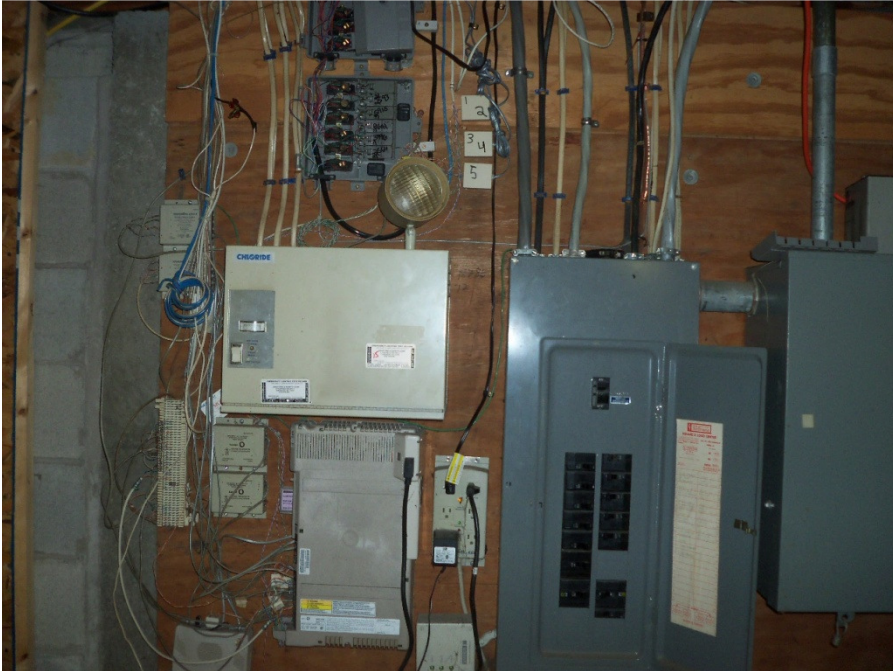
Photo CC-1: Main service and example of Romex wiring
