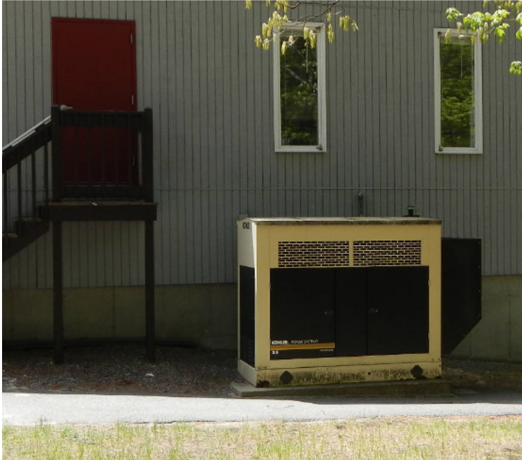
Photo GSC5B: Existing Gas Fired Generator Located on the side of the Building. Windows in this picture are operable.
