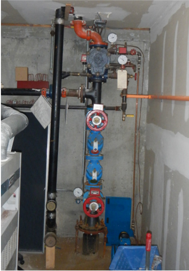
Photo GSC3A(1): Existing Incoming Fire Protection Service. Also shows Existing Sanitary Exit from the Building Propped up by Wood
