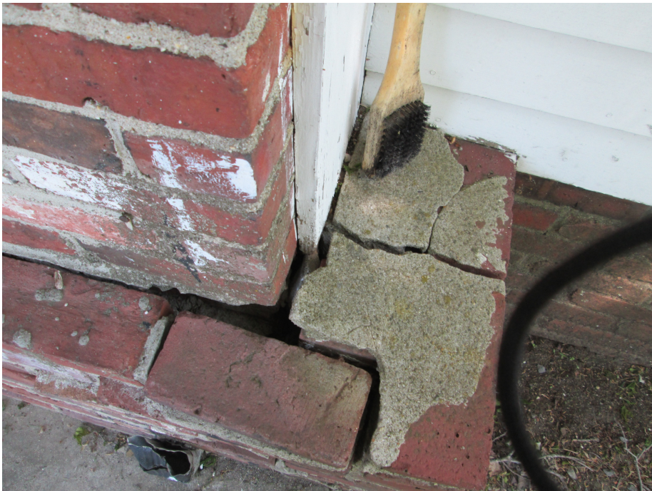
Photo CC7C: Portion of deteriorated brickwork at front elevation.
