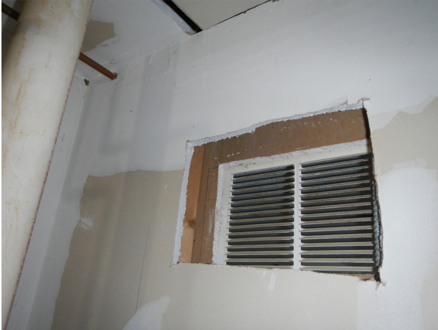
Photo GSC29: Unprotected opening in fire-rated wall construction
