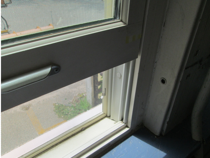
Photo PS8B: Entire building has been retrofitted with new energy saving insulated glass windows.
