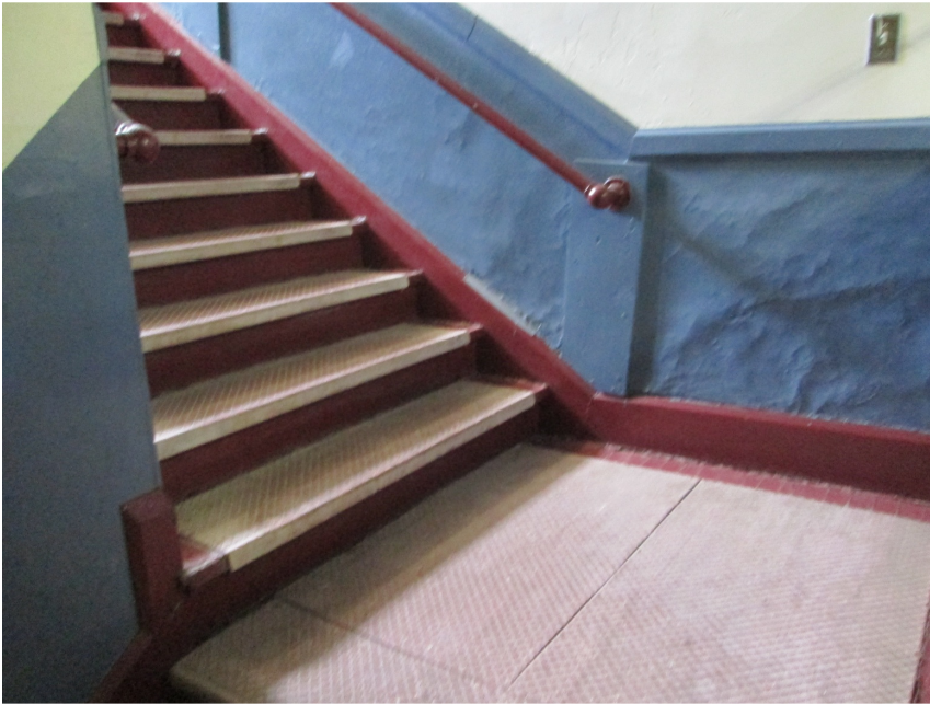
Photo PS4E: Non-compliant features include railings, varying riser heights, and projected stair nosings.
