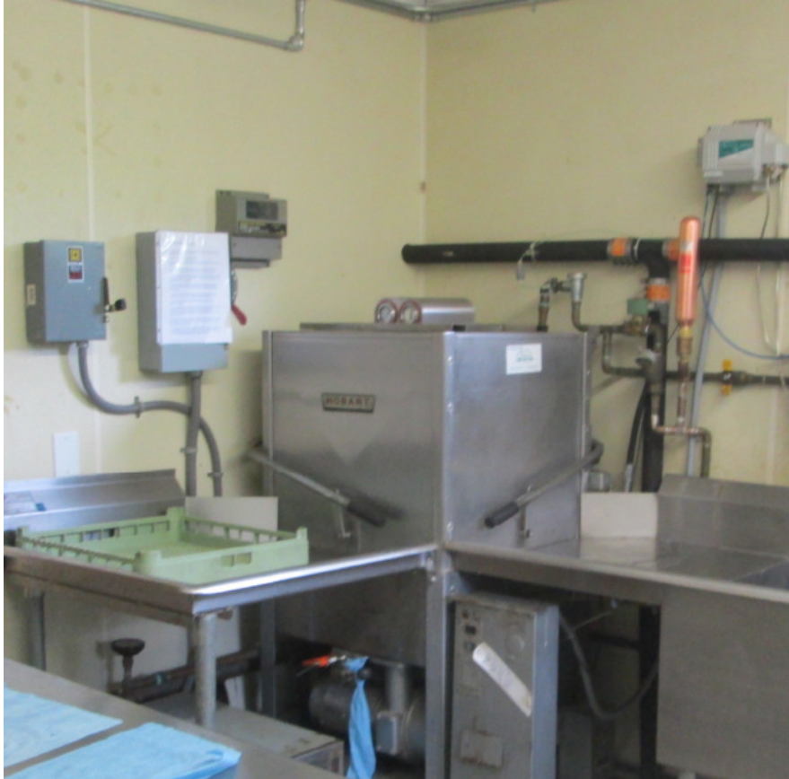
Photo CC7A: Existing Dishwasher without Type II hood.
