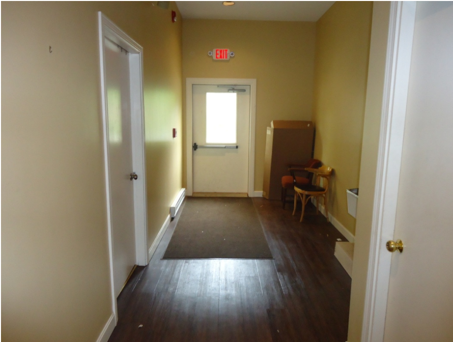
Photo CC4H: Raised threshold at exit door results in tripping hazard. Inaccessible knob door hardware is typical.
