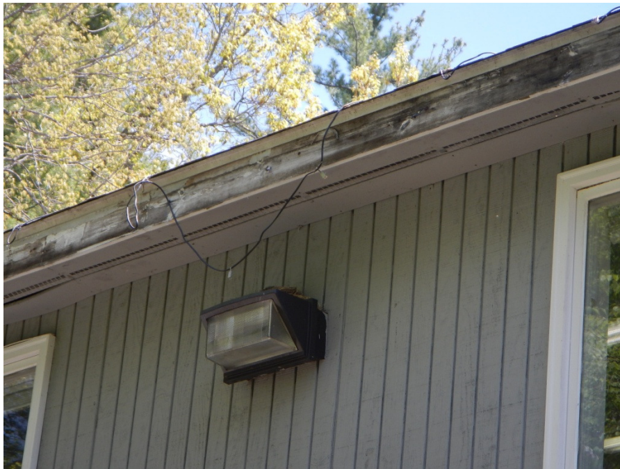
Photo GSC31: Deteriorated wood fascia trim and soffit Loose snow melt wiring system
