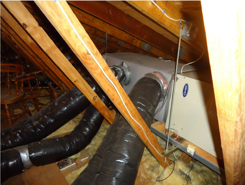
Photo CC7E: Approximately 8 inches of fiberglass insulation at ceiling plane within attic space.
