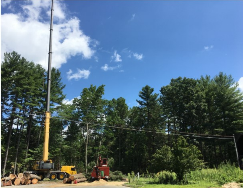
Bitter sweet building demolition
