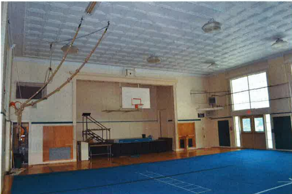
Fig 40. Auditorium space looking south. The stage has wood molding around the masonry opening and an access door on either side. The stage is at the same level as the main floor, but originally was raised 3'-0" and had different wood molding around the opening. The ante rooms on either side of the stage had stairs to access the stage. If renovated for an auditorium space, a larger, raised stage could be designed for this area.
