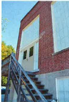
Fig 26. Existing West exit door of Auditorium with Kalwall windows above and at sidelights
