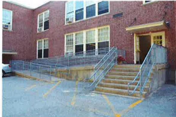
Fig 25. Stair and Accessible ramp added by the Carell Group in 1997
