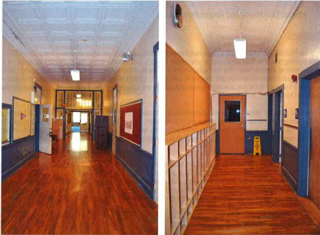
Fig 34. View of the main corridor to the auditorium on the first floor. Note the 8-lite transom panel above the doors. Fig 35. View of the north corridor on the first floor. The wall at the end of the corridor originally had two doors in to the classroom. Also note the exposed electrical wires running along the top of the wall and door.
