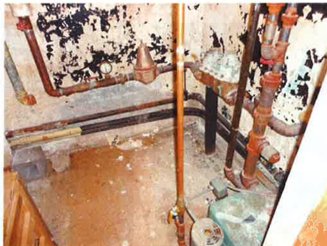
Fig 13. Water service entering front of building in basement
