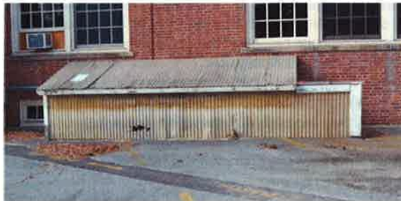
Fig 30. South concrete stairs leading to basement. Fig 31. Other south concrete stairs leading to basement. This enclosure is recommended to be removed and replaced.
