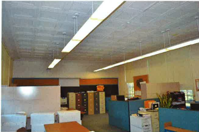
Fig 38. Classroom at Second floor.
