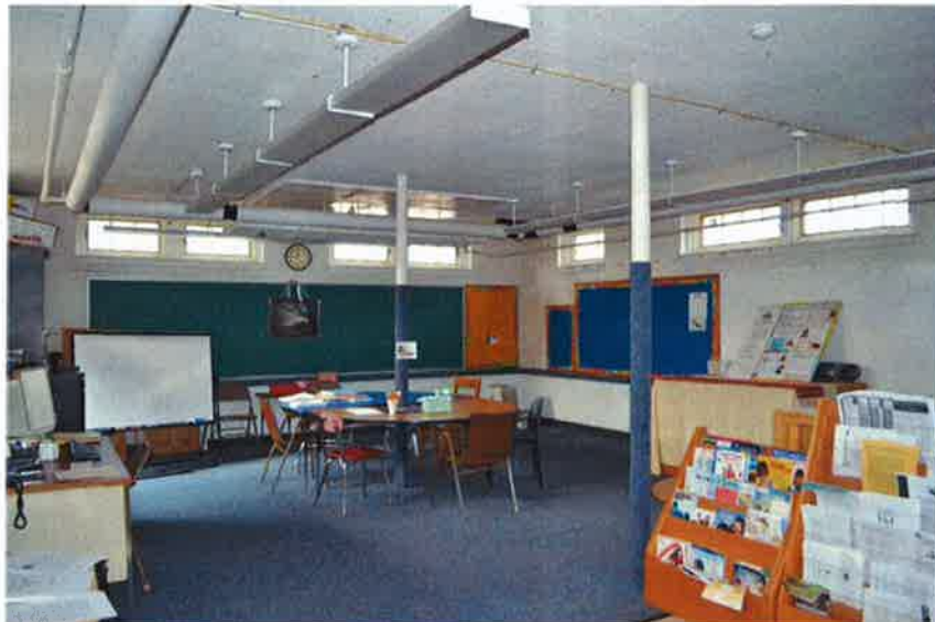
Fig 36. Classroom at basement floor. Note that the window sills are 7'4" from the floor, yet still provide a substantial amount of natural light in the classroom.
