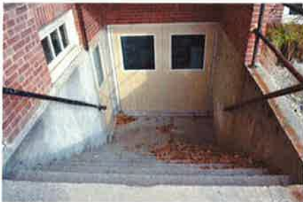
Fig 30. South concrete stairs leading to basement. Fig 31. Other south concrete stairs leading to basement. This enclosure is recommended to be removed and replaced.
