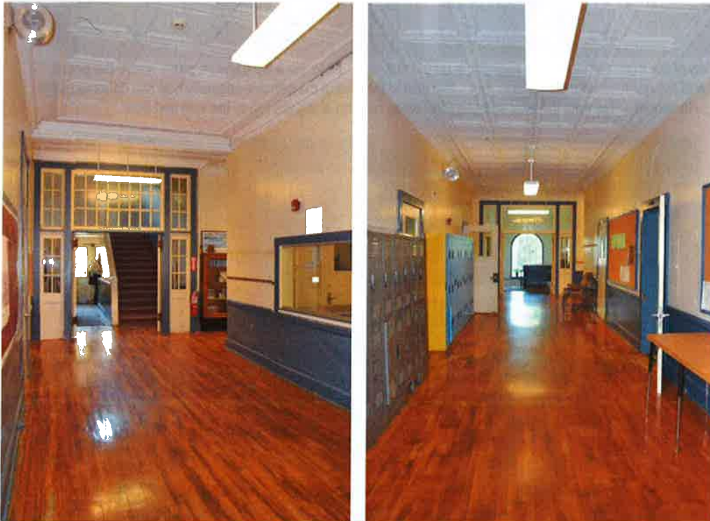
Fig 32. View of East entrance vestibule and stair on the first floor.
