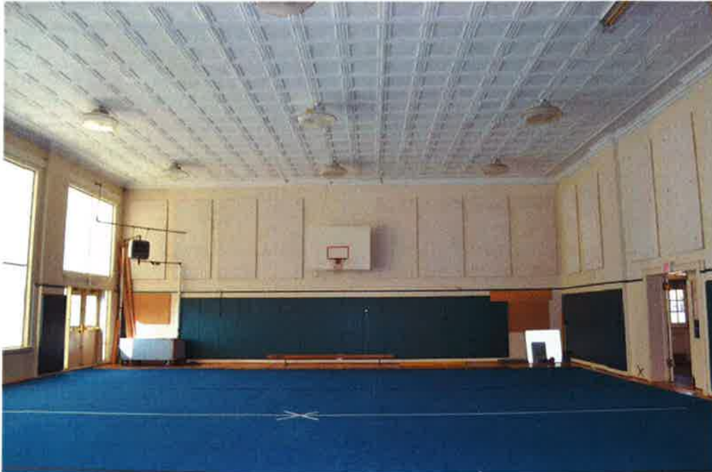
Fig 39. Auditorium space looking north. The walls are exposed brick with the 7' dado, but originally had smooth, terracotta tiles on them.
