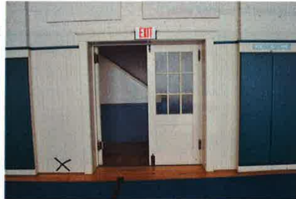
Fig 41. View of dado at corridor wall on first floor. Note the delamination of the material in the dado panel.
