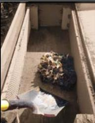
SEDIMENT, LEAVES, AND GRASS CLIPPINGS TRAPPED INSIDE THE CHAMBER ARE EASILY REMOVED BY THE LANDOWNER WITH A SHOVEL. THE DROP-IN FILTER WALL CAN BE EITHER SWEEPED CLEAN OR RINSED WITH A GARDEN HOSE TO MAINTAIN OPTIMAL FILTRATION CAPACITY.
