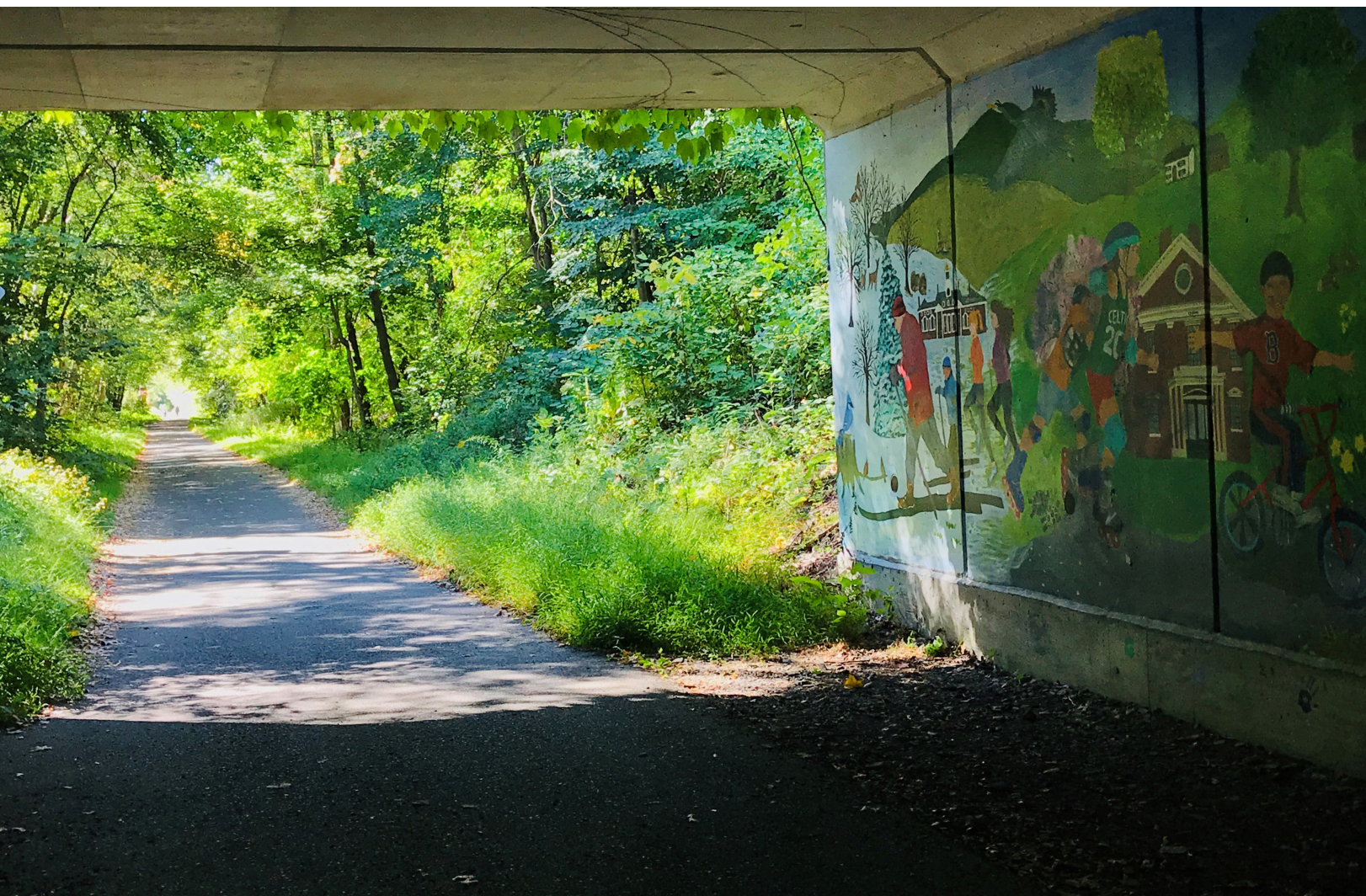
Graphic 3.3.1 Tunnel on the Nashua River Rail Trail. Photo by Lorayne Black.
