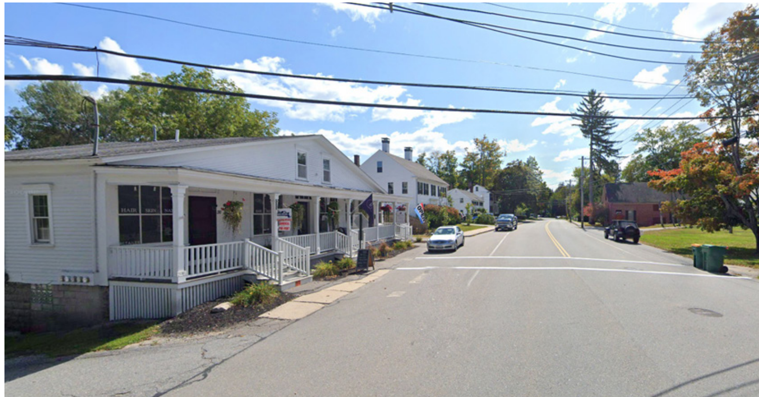
Graphic 4.9. Groton’s sidewalks near businesses are often uneven, narrow, and poorly connected, if present at all. Improvements would allow people to access businesses in the Town Center more safely, such as in this area of Hollis Street. Source: Nitsch Engineering
