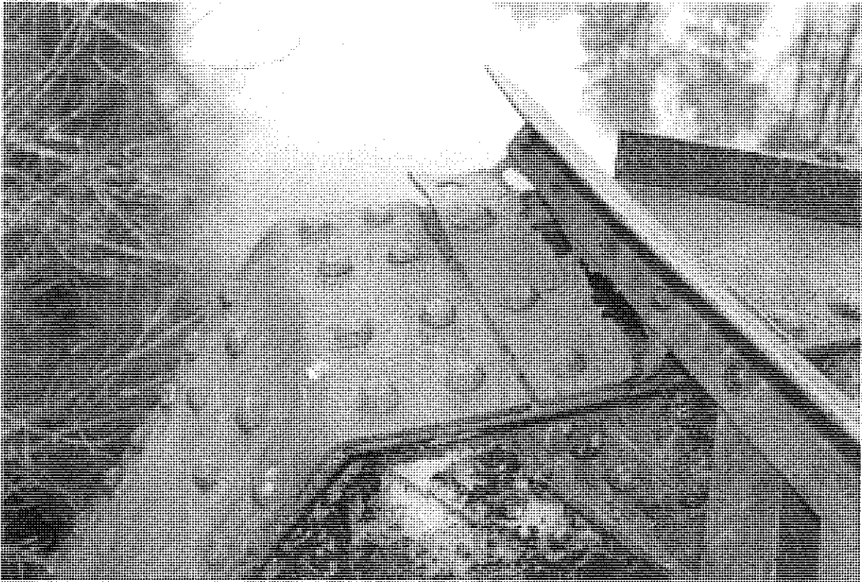
Photo 5 – Corroded Brace Connection and Hole in Top Flange Plate at Portal Connection at N2 Top Chord
