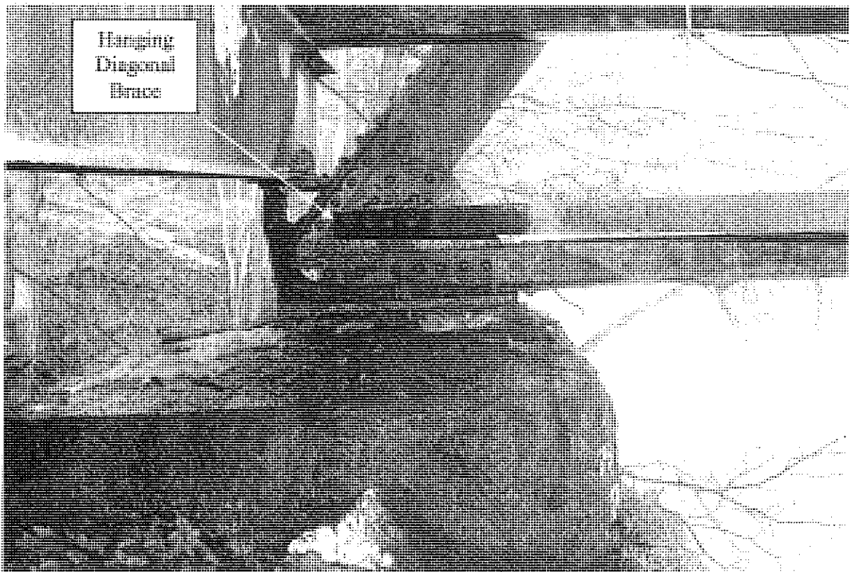
Photo 14 – Broken Gusset Plate and Hanging Diagonal Brace at N1
