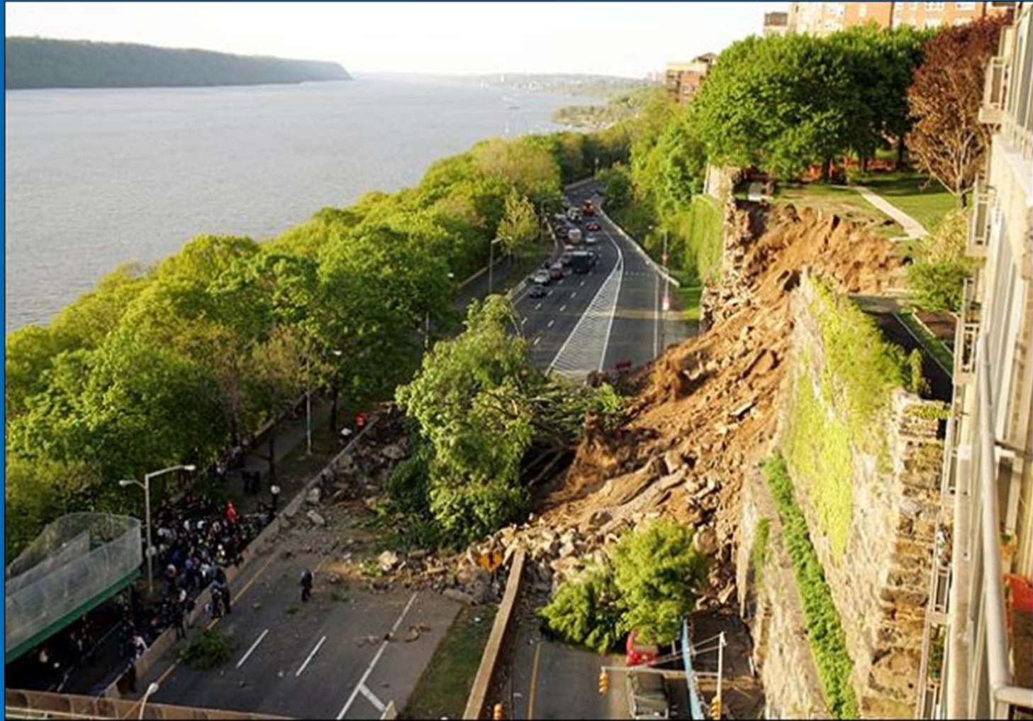
Retaining wall slump along Hudson River Parkway, New York City
