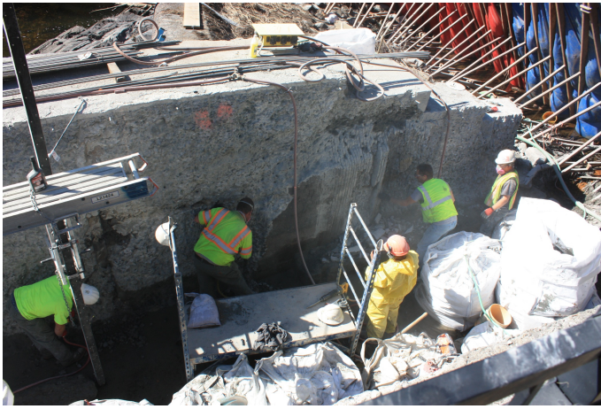
Ongoing chipping on east side of wall
