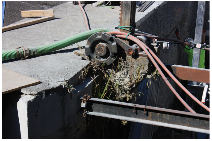
Concrete support for gearbox needs repair.
