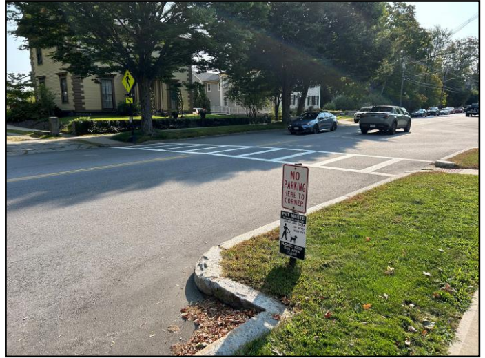
Small bump out in front of town hall
