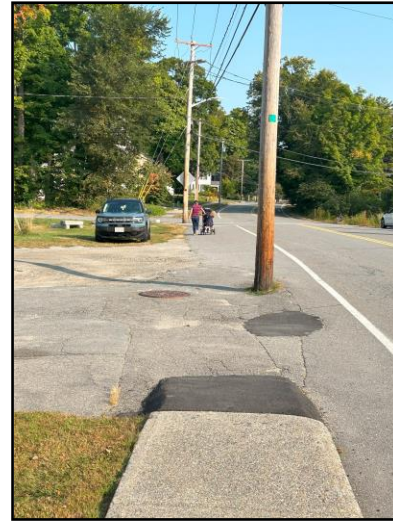
Hollis Street – missing sidewalk link
