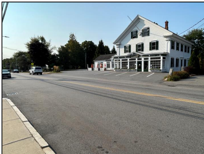
Wide curb cut at Filho's
