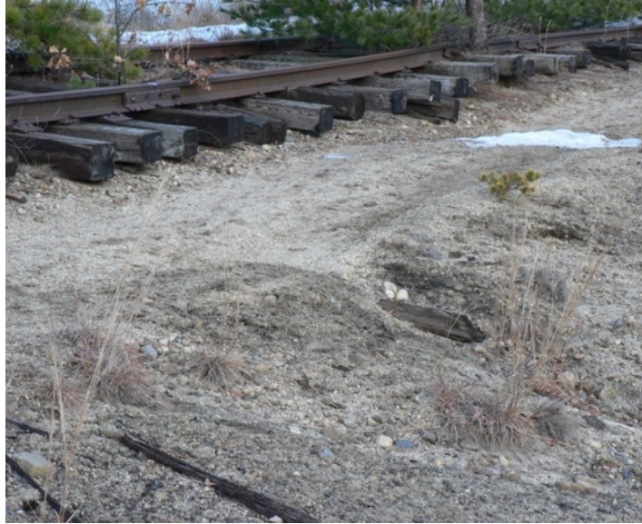
Figure 4: Eroded sub base between Sterilite and self-storage facility. Additional ballast is needed in this area.
