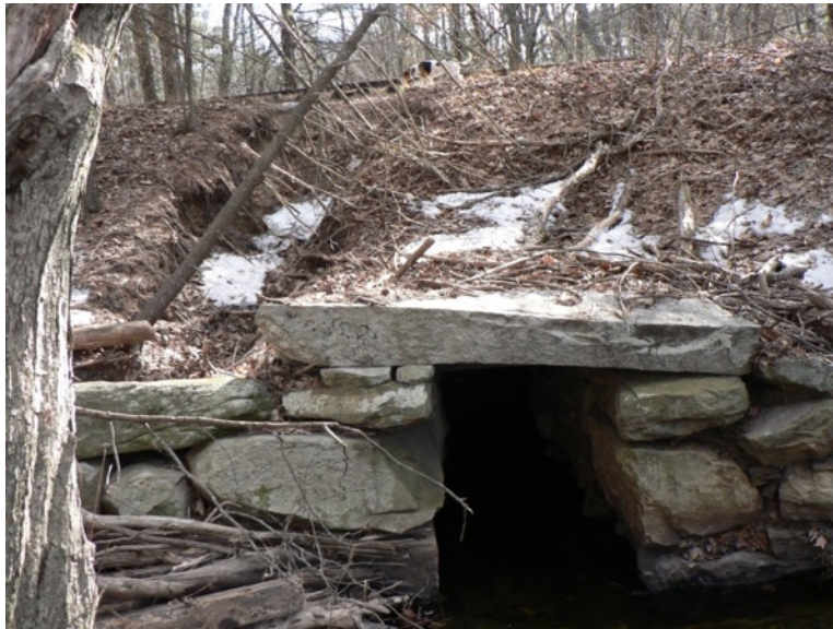
Figure 6: Washed out area above culvert No. 43.89 east of Shepherd's in Townsend
