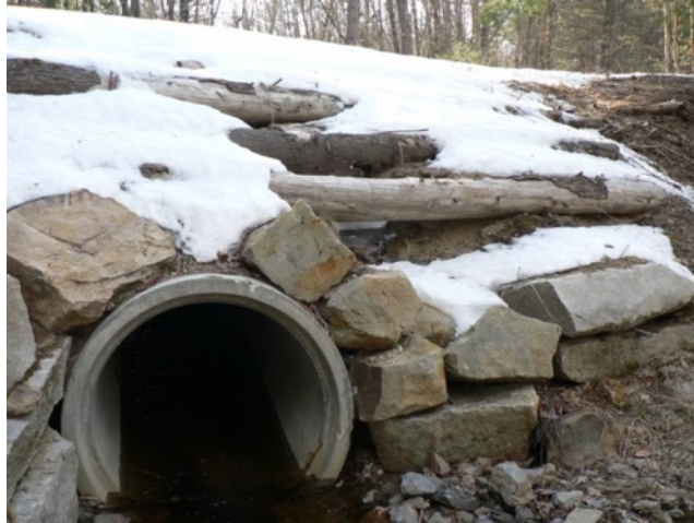
Figure 5: Erosion above culvert No. 42.37 east of Harbor Village
