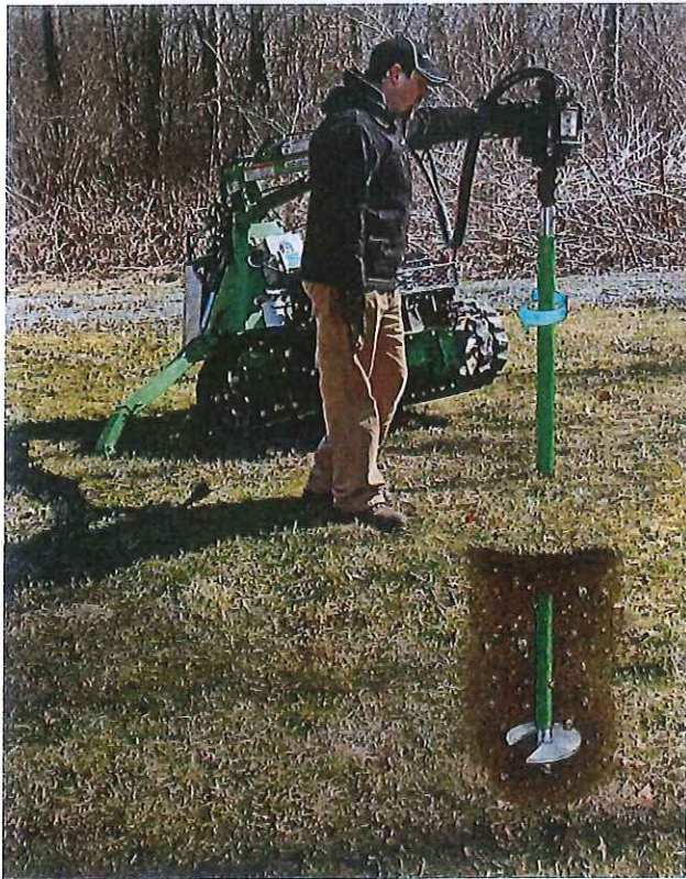
Figure 10. Helical pier and installation example
