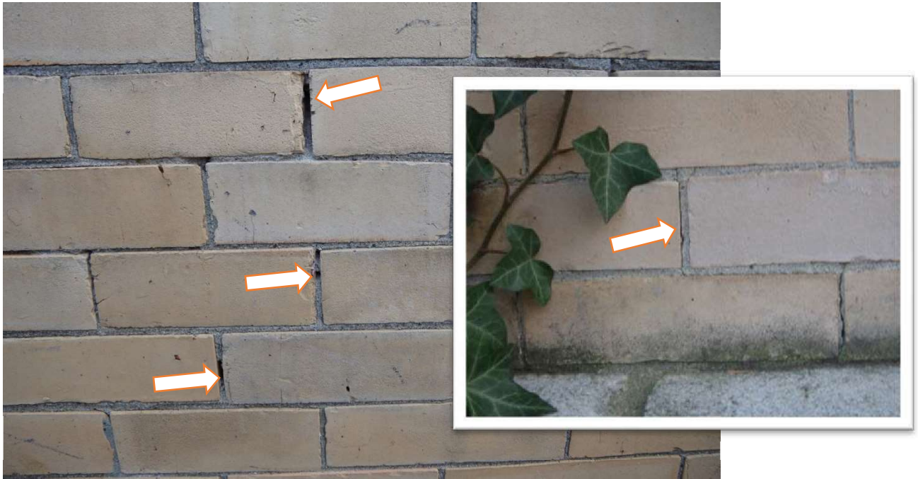
Photo 52 – The exterior mortar joints have a concave profile with a primary mortar type that appears to be original mortar. The secondary mortar type appears to be repair mortar. Overall, the original mortar appears to be in fair condition, however, isolated areas of open or debonded mortar and step cracking were observed.
