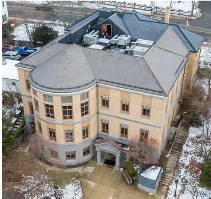
Photo 60 – The above-grade exterior masonry walls are primarily constructed of a brick or precast concrete veneer and CMU backup wall. At the west elevation, the lower level is a coursed precast concrete veneer with precast concrete water table. The middle and upper levels are brick veneer and include precast concrete string courses, corbelled brick string courses, and a corbelled brick and fiberglass cornice.
