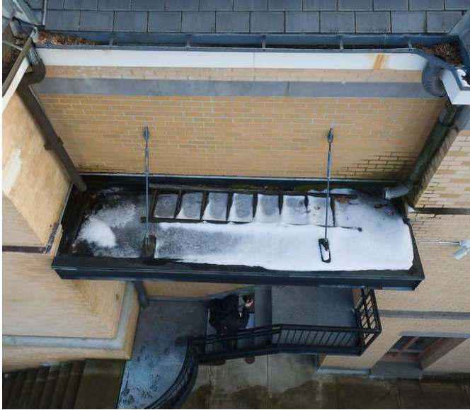
Photo 47 – Other isolated roof areas and canopies were observed to have single-ply elastomeric roof systems located at the north and south elevations. At both locations, the roof membrane terminates with a termination bar and sealant.
