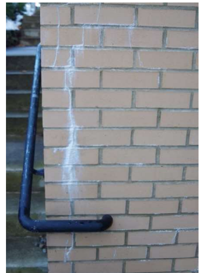
Photo 61 – The primary area of the exterior brick veneer is laid in a running bond and concave mortar profile. Secondary areas are laid in a Flemish or basket weave bond. Overall, the brick units were observed to be in good condition with isolated areas of deterioration including step cracks and efflorescence.
