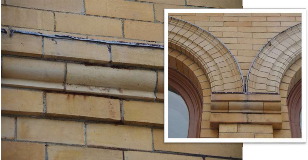
Photo 54 – Partial view of corbelled brick string course and roman arches. Weathered lead coated copper flashings were observed above the corbeled brick string course and roman arches. The string course has a concentrated area of mortar deterioration along its entire length.
