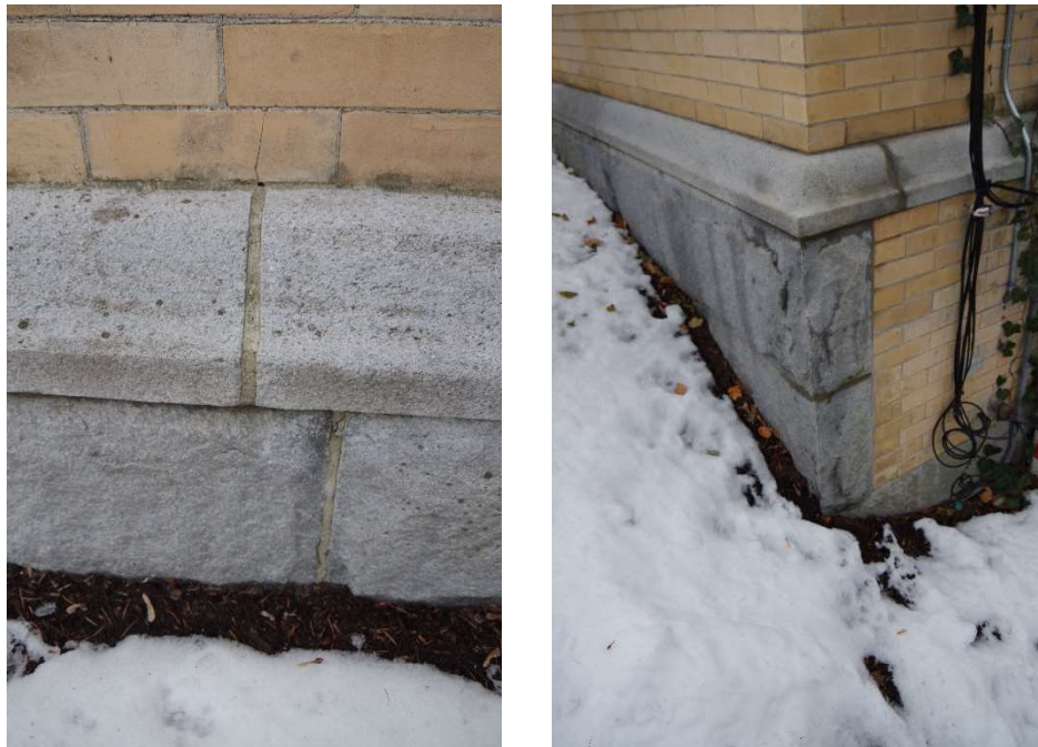
Photo 53 – Partial view of coursed granite water table and foundation. Overall, the granite and mortar appeared in good condition. The granite water table has a concentrated area of mortar deterioration at sky facing bed joints.
