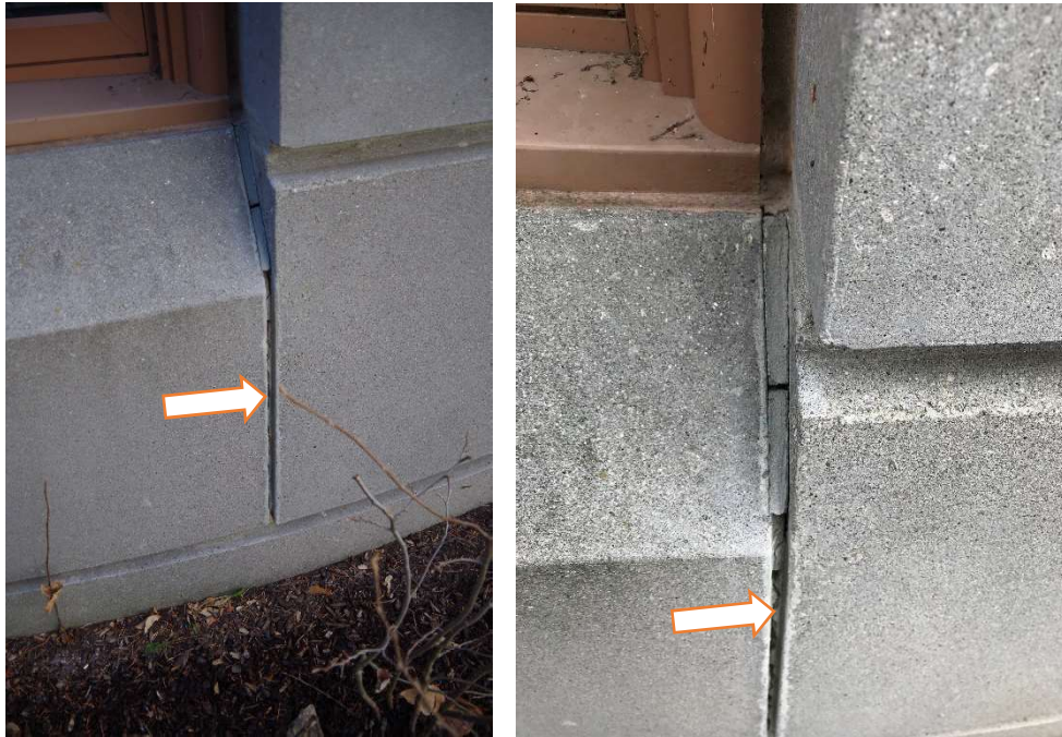
Photo 62 – Isolated areas of cracked or open mortar joints were observed at the areas of precast concrete veneer, particularly at the window sills.
