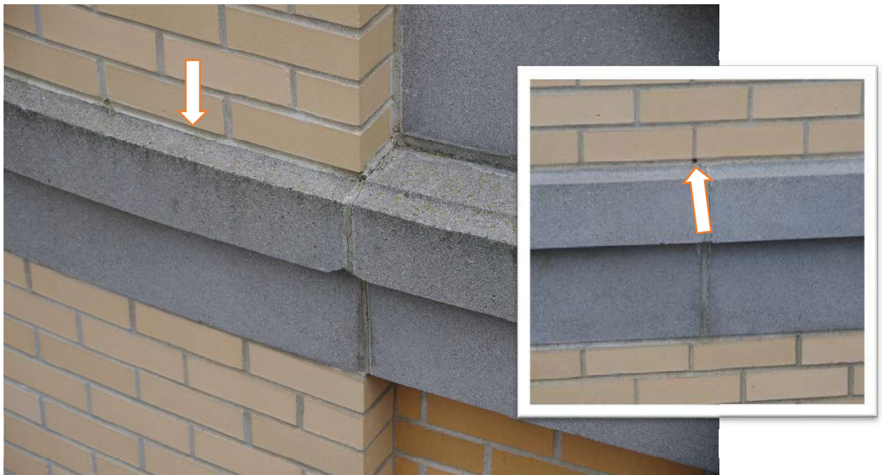
Photo 63 – Sheet metal flashings shown on the original design drawings are not visible from the exterior and may be embedded within the masonry mortar joints at typical locations throughout the building including above window heads, stringer courses and transitions between the brick masonry and precast veneer. Weep holes were observed above the precast stringer courses, indicating likely flashing locations.
