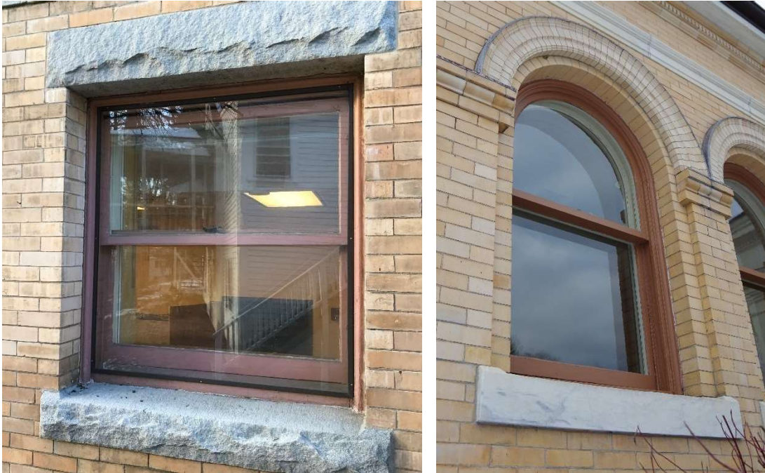
Photo 58 – Lower level windows appear to be wood, single-glazed, double-hung units with exterior painted wood brick mold. Window hardware appeared in poor condition and window sashes did not appear locked. Fixed exterior storms were observed at three lower level windows on the south elevation, for additional insulation and weather protection. Six upper level windows are wood, single-glazed, single-hung arch tops with exterior painted wood brick mold. Interior storm windows were installed at these window units for additional insulation. Exterior paint coatings appeared to be weathered and beginning to fail in several locations. Failed exterior perimeter sealants were observed at most locations.
