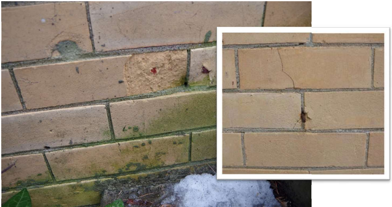
Photo 51 – The exterior brick masonry wythe is laid in a running bond. Isolated areas of cracked, spalled, and delaminated brick were observed throughout. Efflorescence, metal anchors, and vegetative growth were also observed.
