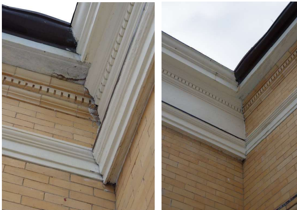
Photo 57 – Partial view of entrance portico's wood entablature transitioning to the stone and brick entablature of the east elevation. This is also where the wood gutter with copper lining transitions to the hanging copper gutter.
