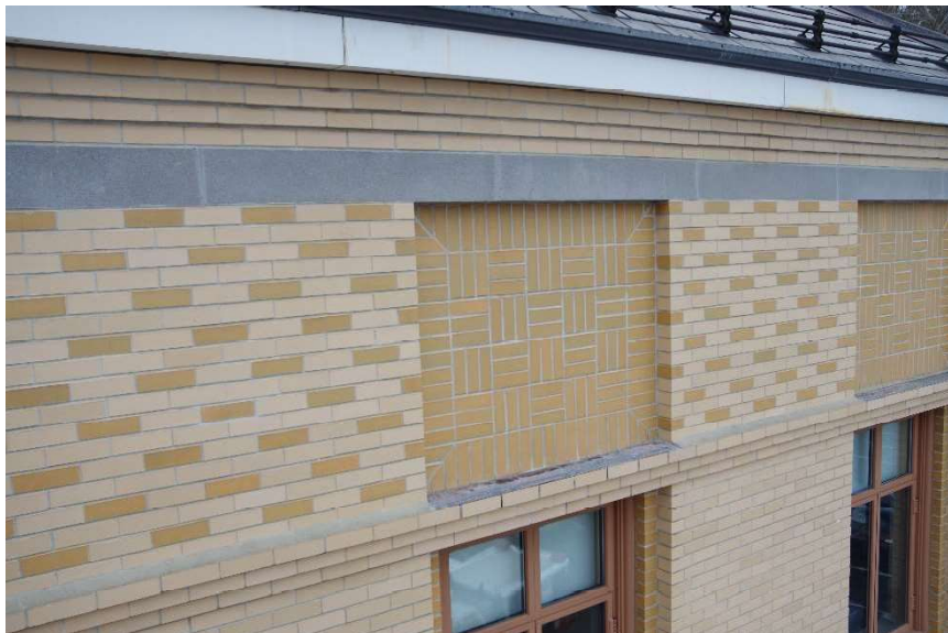
Photo 61 – The primary area of the exterior brick veneer is laid in a running bond and concave mortar profile. Secondary areas are laid in a Flemish or basket weave bond. Overall, the brick units were observed to be in good condition with isolated areas of deterioration including step cracks and efflorescence.
