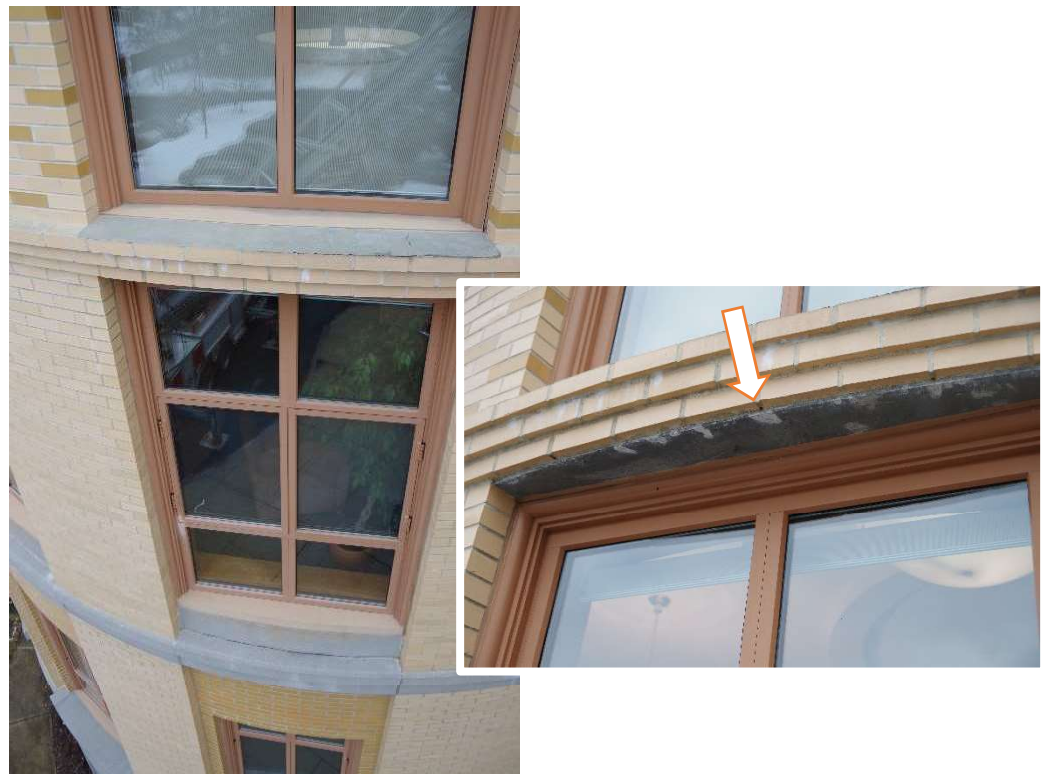
Photo 65 – Aluminum framed windows consist of fixed and project out casement operation with insulated glazing. Embedded steel lintels to support the masonry veneer components above the window were not partially visible and consist of galvanized steel. Weep holes and moisture stains observed above lintels appear to indicate the presence of embedded flashings.
