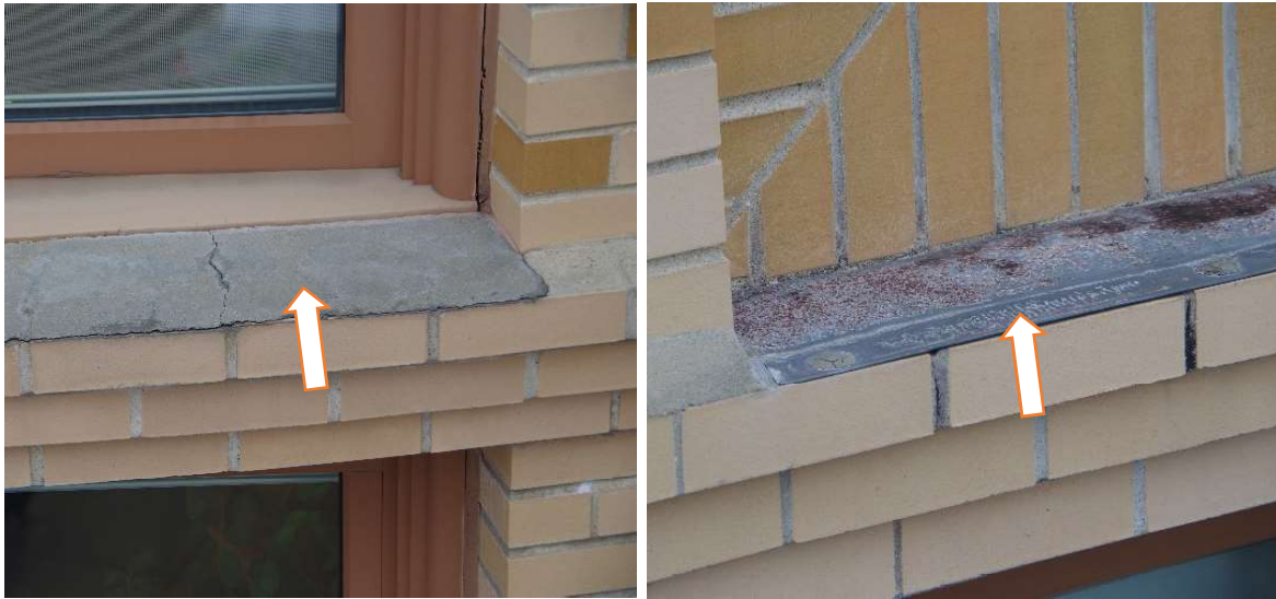
Photo 64 – Mortar cants/washes are installed above the corbelled brick stringer courses in several locations to shed water off of the horizontal surfaces. At isolated areas, this mortar cant/wash is cracked or spalled. Other areas were observed to have lead coated copper flashings atop the corbelled masonry in lieu of the mortar wash.
