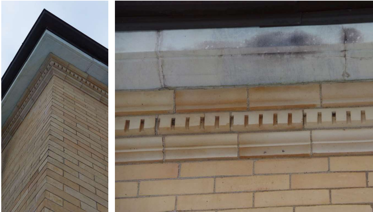
Photo 56 – Partial view of marble cornice where cracked and discolored stone was observed. Isolated areas of mortar deterioration were observed at both the marble and terra cotta elements of the cornice.
