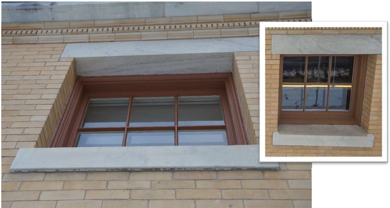
Photo 59 – Upper level wood, single-glazed, clerestory window with six lights and exterior painted wood brick mold appear to be in fair condition. Interior storm windows were installed at these window units.
