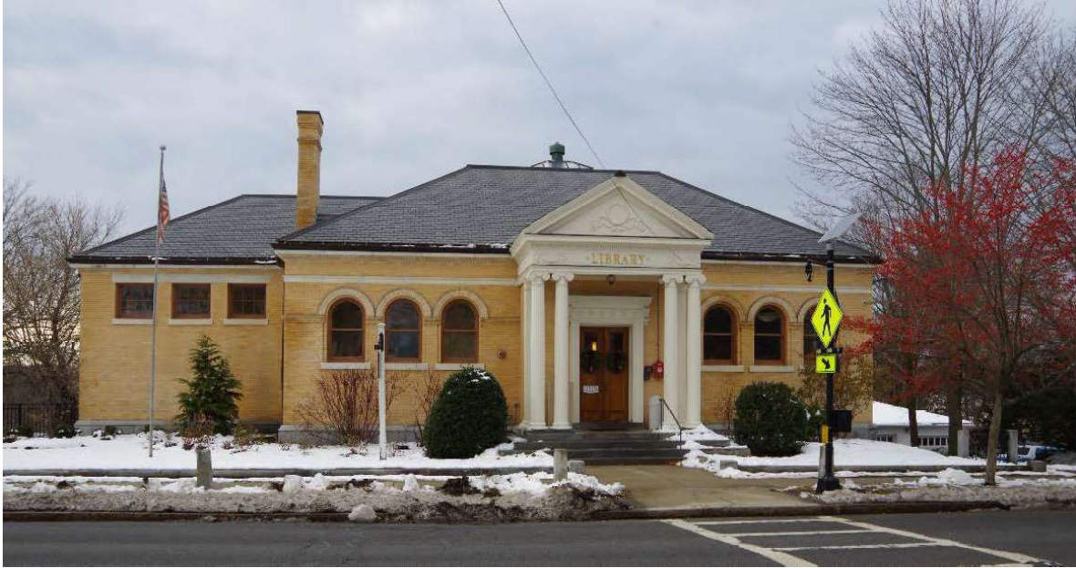
Photo 50 – Overall view of the east elevation. At the original structure, the above-grade exterior masonry walls are primarily constructed of 3-wythes of brick masonry. The main upper level elevation includes coursed granite water table, corbeled brick string course, brick roman arches, marble string course, and terra cotta and marble cornice. Lower level window openings (not shown) have granite sills and lintels. Upper level window openings have marble sills and either marble lintels or brick roman arches. The painted wood entrance portico appears to be in fair condition.
