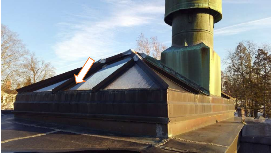
Photo 49 – Partial view of hipped skylight and edge metal at copper roof. Previous flashing repairs were observed at the skylight. The arrow indicates failed glazing seals that were observed. It also appears that some of the glazing has been previously replaced.
