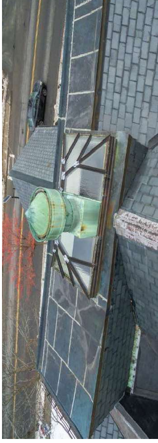
Left: 1893 library copper gutters, downspouts, & windows
