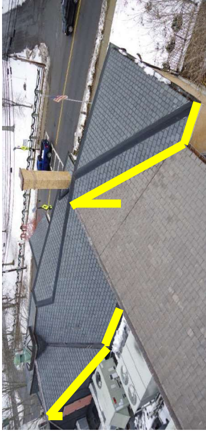
Above: Approximate demarcation of 1893 Slate Roof from 1999 addition.
