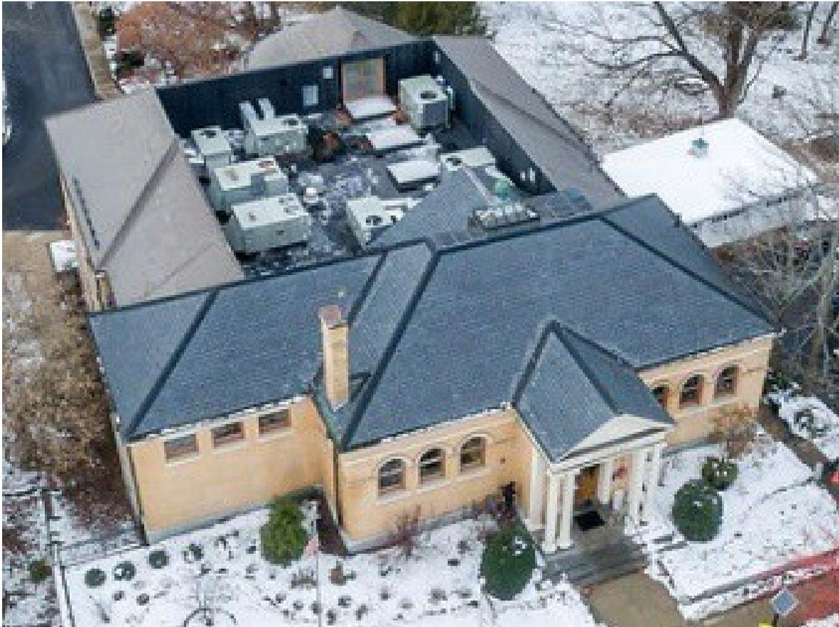
*View of the 1893 library slate roof, with elastomeric membrane (EPDM) roof and HVAC area behind, and 1999 sloped roof to the rear.*
