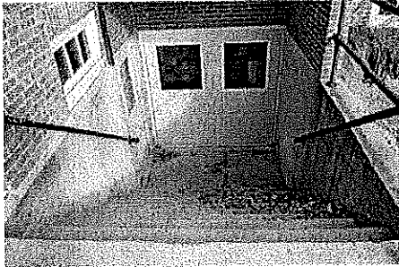
Fig 31. Other south concrete stairs leading to basement. This enclosure is recommended to be removed and replaced.
