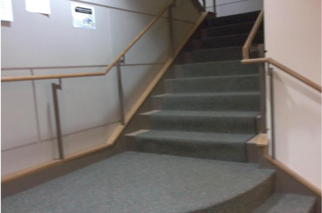
*The Team found that the stairs (including the handrails) were designed and built in compliance with the ADA.*
