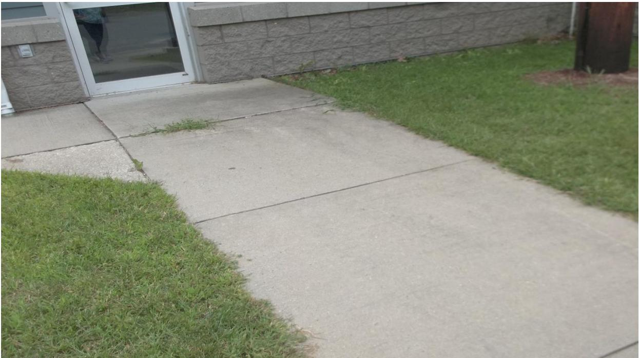
*The ADA team found that there are cracks and weeds that have formed on the sidewalk that exceed  $\frac{3}{4}$  inch. We recommend these be patched with fresh concrete with a suggested target date of December/2018.*
