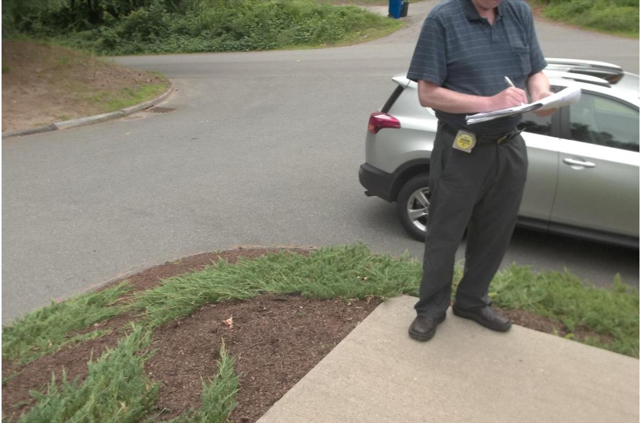
*In order to achieve better accessibility and safety, we recommend that a protection railing be installed on the Fire Station walkway. This may help prevent visitors and staff from falling off the hilly area adjacent to the concrete walkway.*
