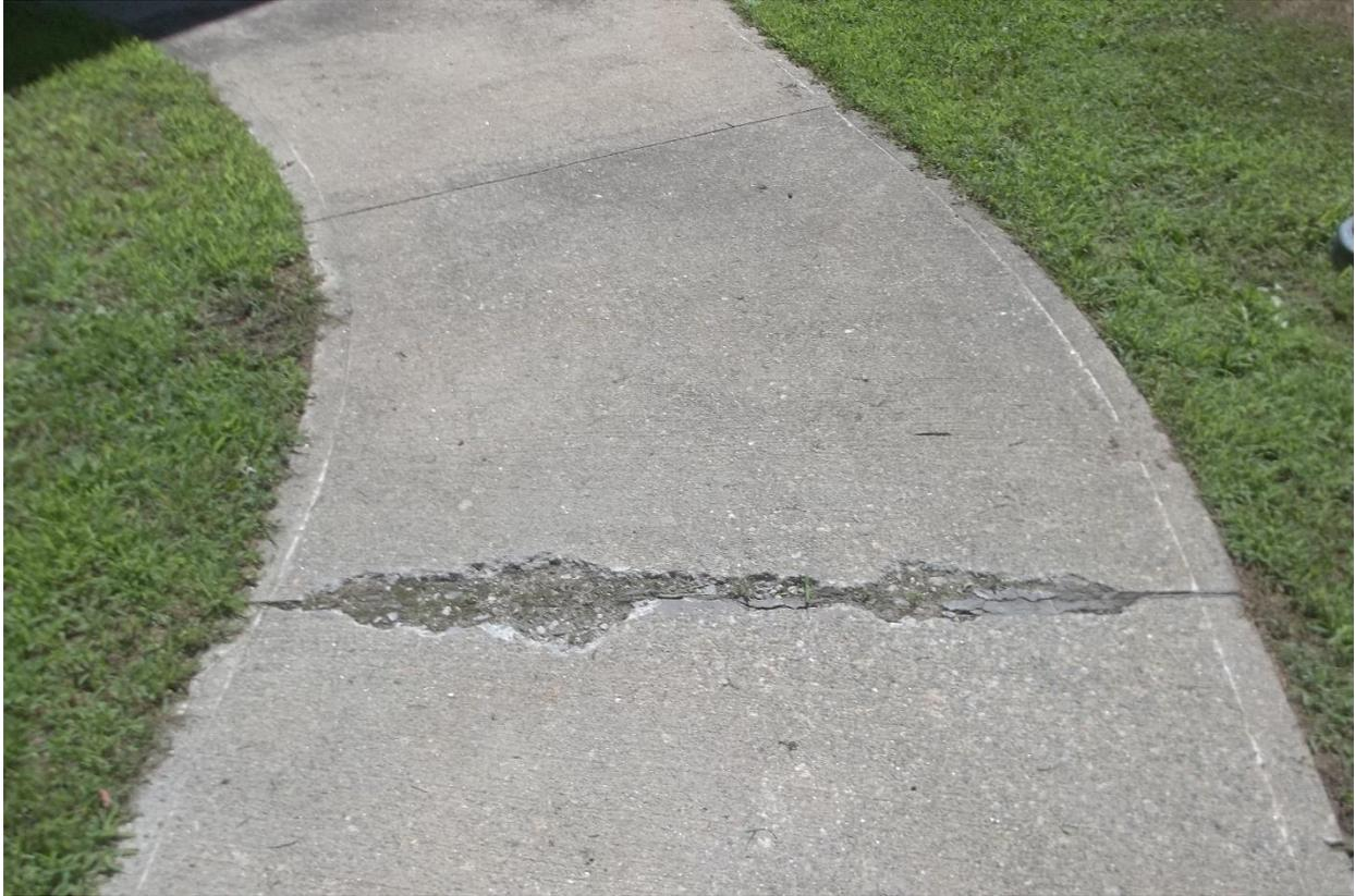
*The concrete walkway to the accessible entrance was found to have three sets of cracks that each exceed  $\frac{3}{4}$  inches. We recommend these cracks be repaired to allow for an even leveled (stable, firm, and smooth) pathway to the accessible entrance. This is due to the effects of natural wear and tear.*
