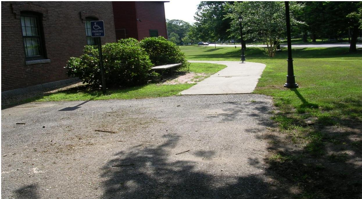
*The first Legion Common ADA transition Plan action step is to add a van accessible sign under the HP parking sign already there. Specifically, the Van sign under the ADAAG section 4.6.4, requires that accessible parking spaces be "designated as reserved by an above-ground sign showing the symbol of accessibility. Spaces shall have an additional sign 'Van Accessible' mounted below the symbol of accessibility". In this way, we recommend the town install one van accessible HP parking spot.*
