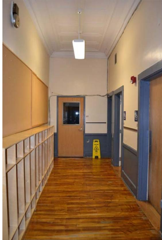
Fig 34. View of the main corridor to the auditorium on the first floor. Note the 8-lite transom panel above the doors.
