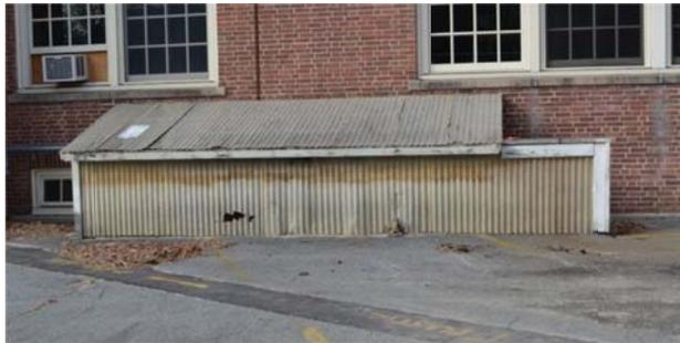
Fig 31. Other south concrete stairs leading to basement. This enclosure is recommended to be removed and replaced.
