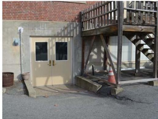
Fig 29. West basement entry, non-compliant ramp
