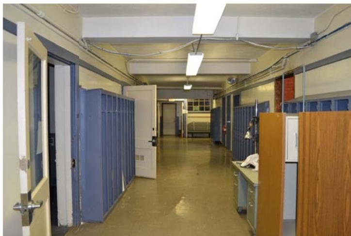
Fig 46. Vinyl asbestos tile in the basement are recommended to be removed.
