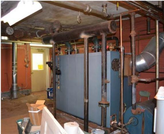
Fig 10. Existing gas-fired boiler in basement.
