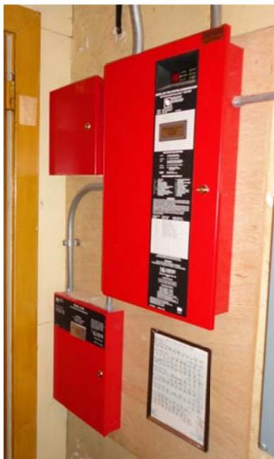
Fig 20. Fire Alarm panel in electrical room in basement.
