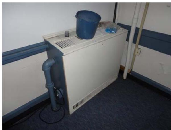
Fig 12. Existing unit ventilator
