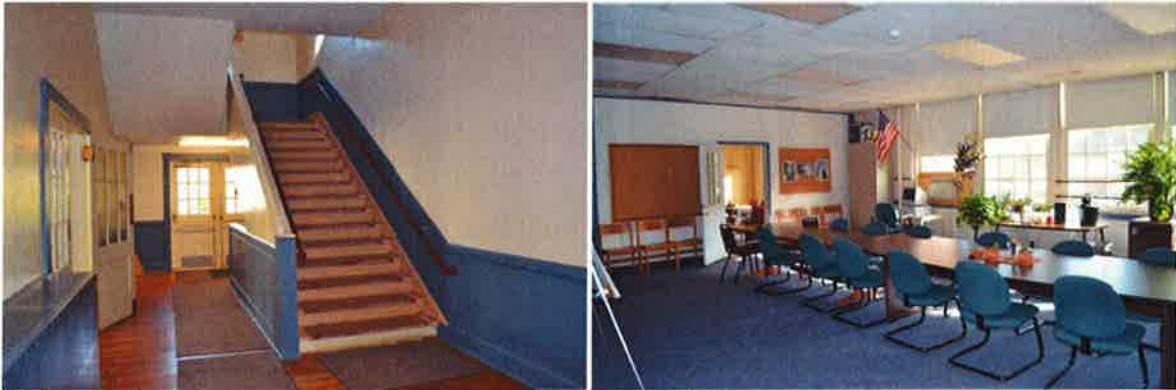
Fig 43. View of metal stair at north entrance. Handrails and a guardrail would be need to bring the stair up to code.
