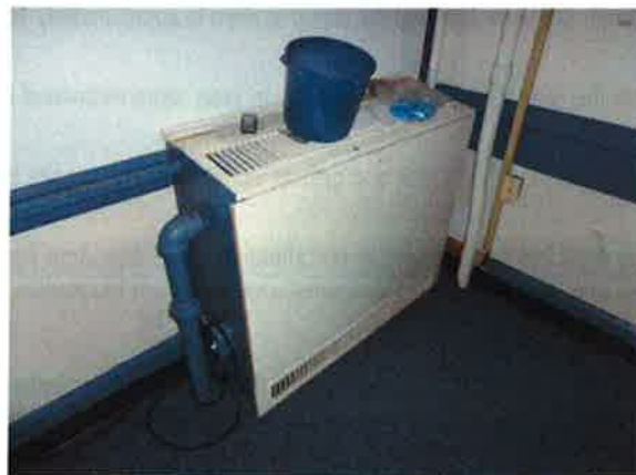
Fig 12. Existing unit ventilator
