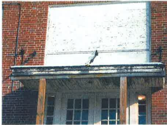
Fig 26. Existing West exit door of Auditorium with Kalwall windows above and at sidelights
