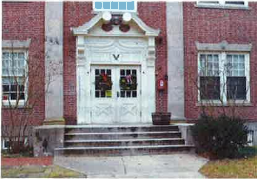
Fig 28. East entry non-compliant stairs
