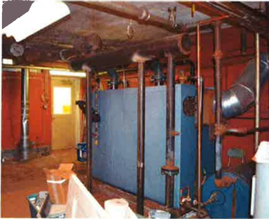
Fig 10. Existing gas-fired boiler in basement.
